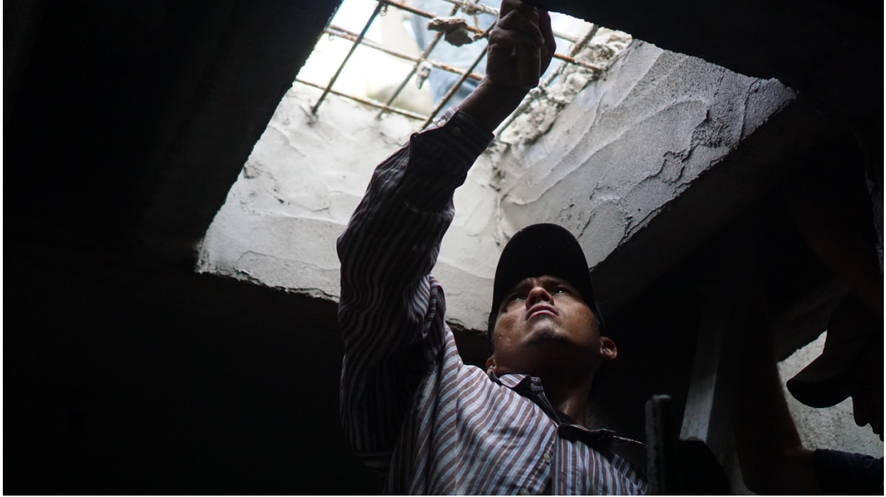
Figure 5.1: Gustavo working concrete in Huixtla, Chiapas
