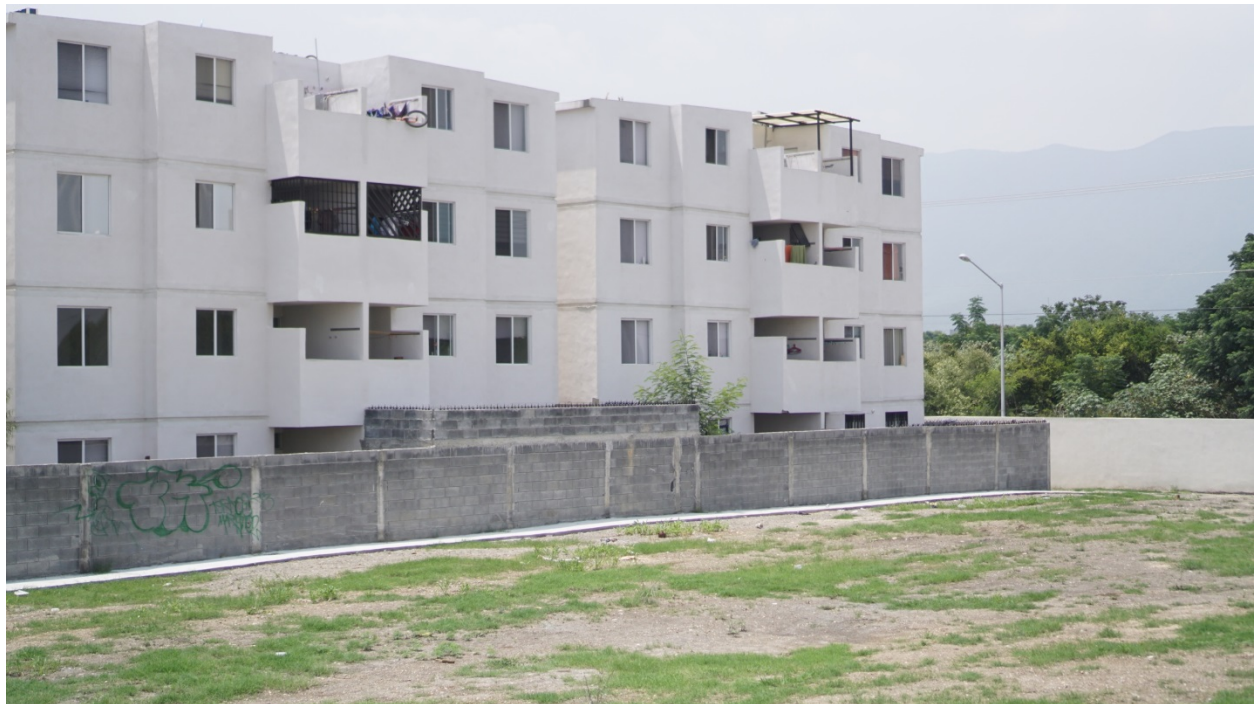
Figure 6.2: Window grates on a suburban apartment complex in Monterrey, Nuevo Leon
