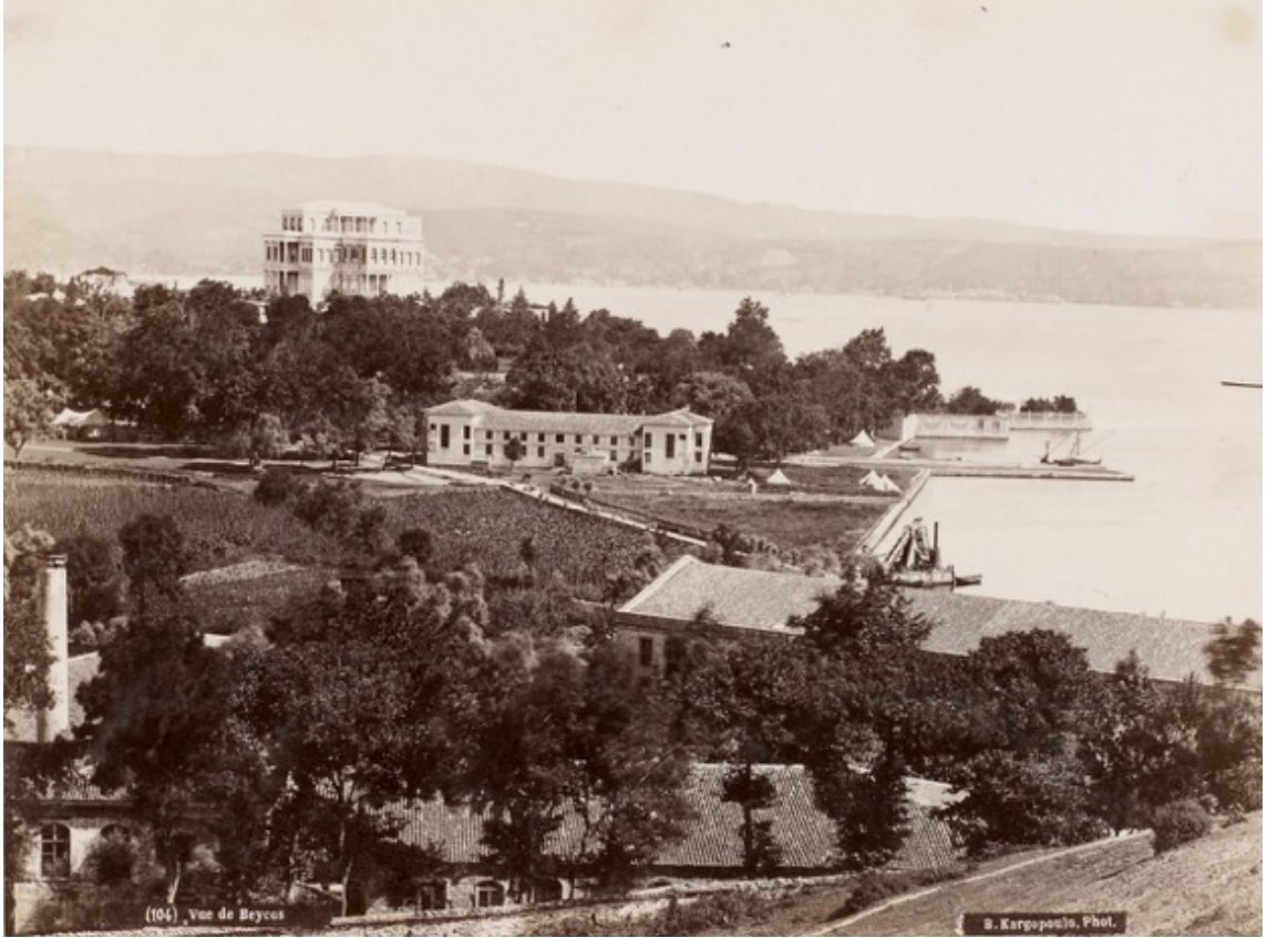
Figure 1.58: “Vue de Beycos” (Beykoz Kasrı) with tents on the shore, B. Kargopoulo Photography, Istanbul University Rare Books Library and Photography Archive, inv. no. 9/631/25.
