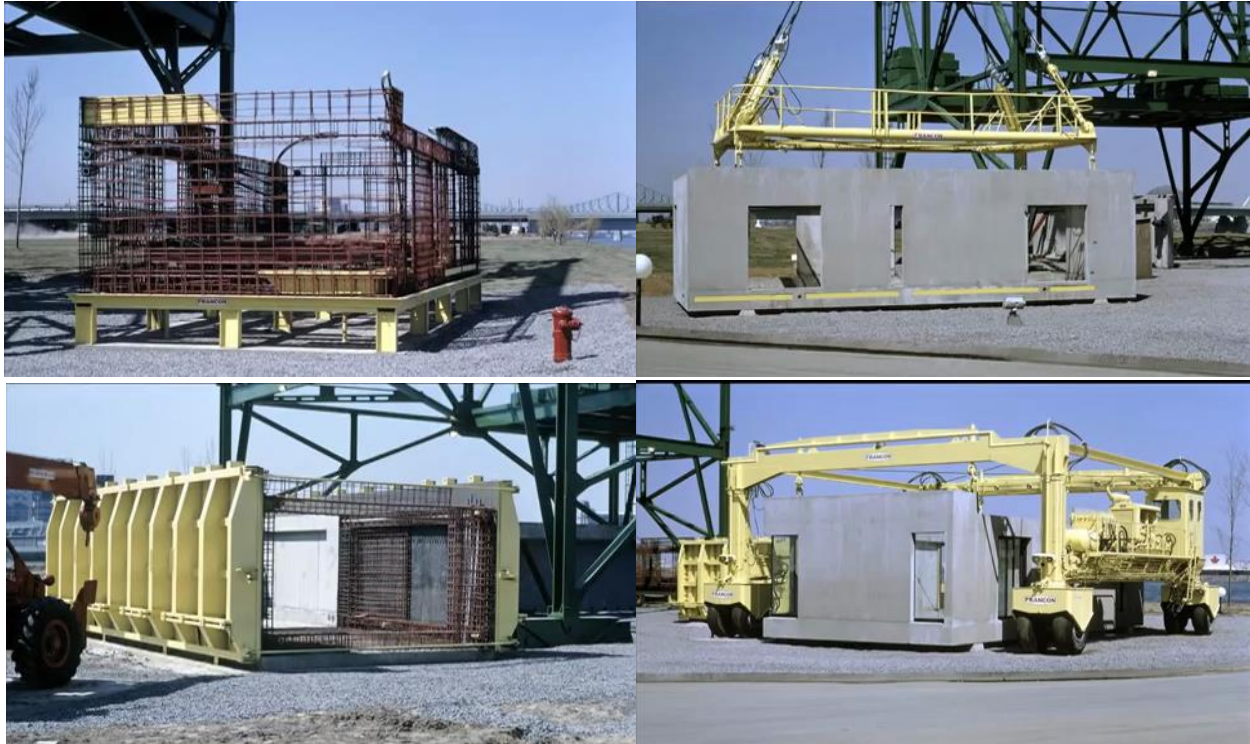
Figure 84: Prefabrication of the apartment units in the manufacturer's site [111]
