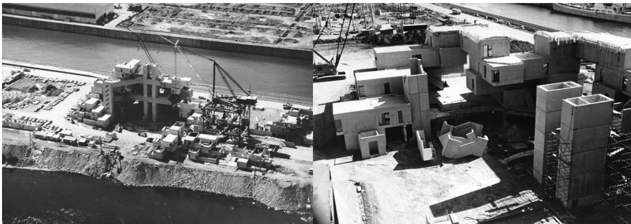
Figure 85: Construction of Habitat 67 [112]
