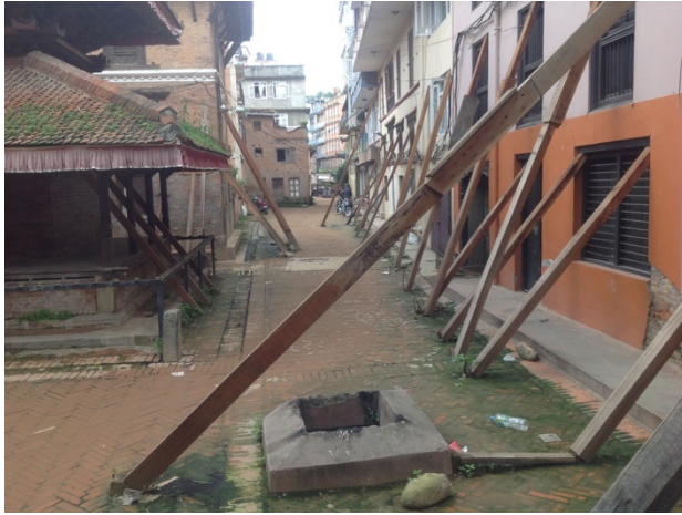
Figure 7: Street in Patan with damaged houses braced, August 2015
