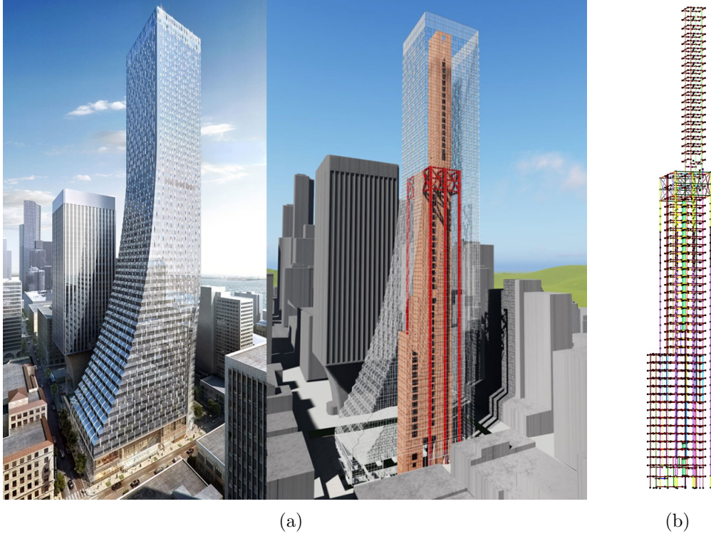
Figure 6.1: Rainier Square Tower. (a) Architectural and structural system rendering of the building (Hilburg, 2018); (b) OpenSees finite element model.
