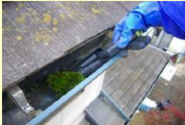
Removal of sediments and washing of inner surface of eaves trough
