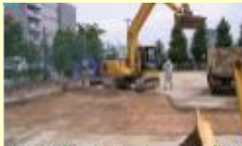
Removal of surface soil of school ground with heavy machine and burying in a pit bored in the ground
