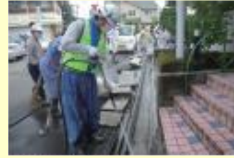
Removal of sediments and washing of Inner surface of road-side ditches
