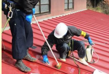
Brushing and wiping of rust or stain on roof surface
