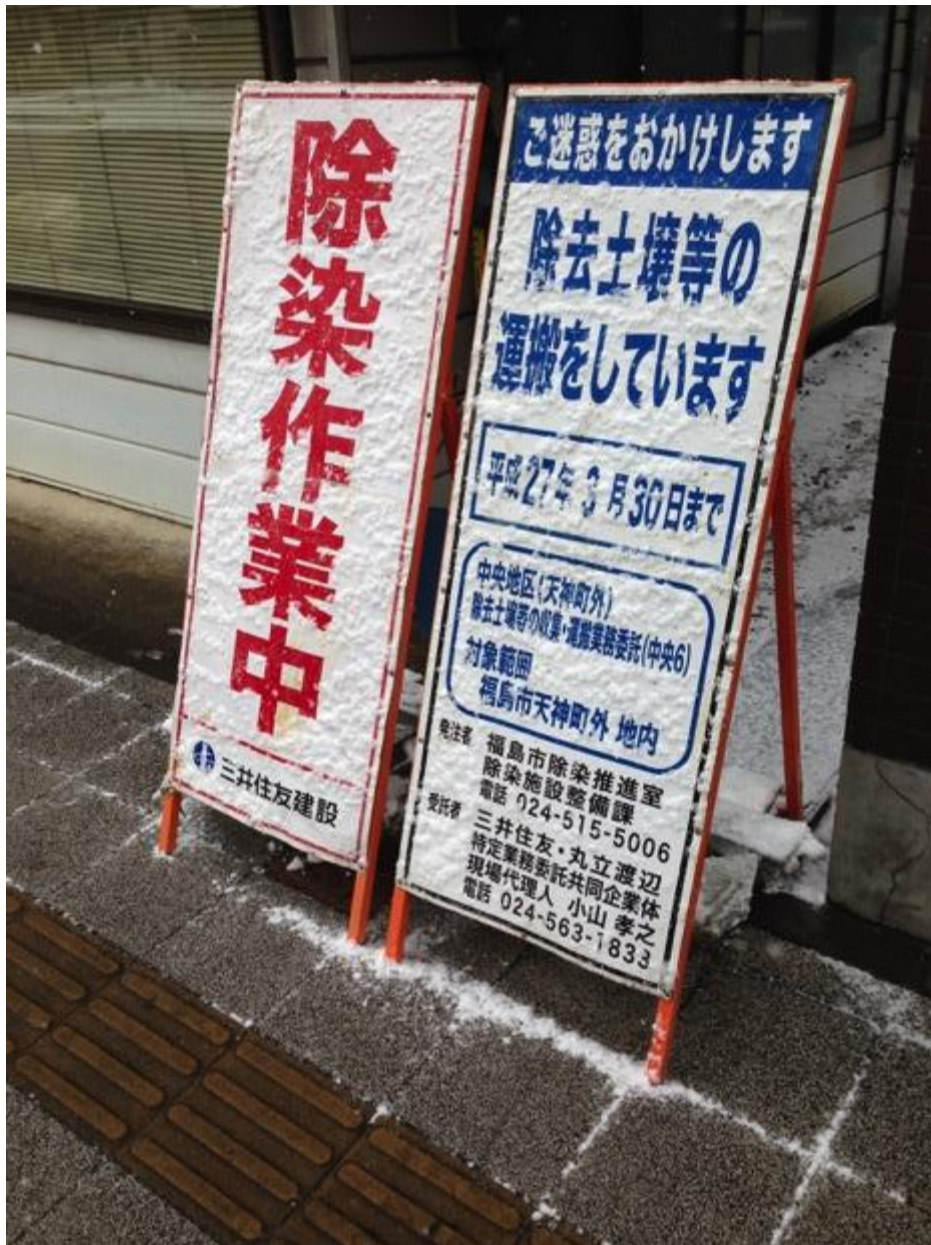
Figure 3.16 “Decontamination in progress” signs on sidewalk in Fukushima City.
