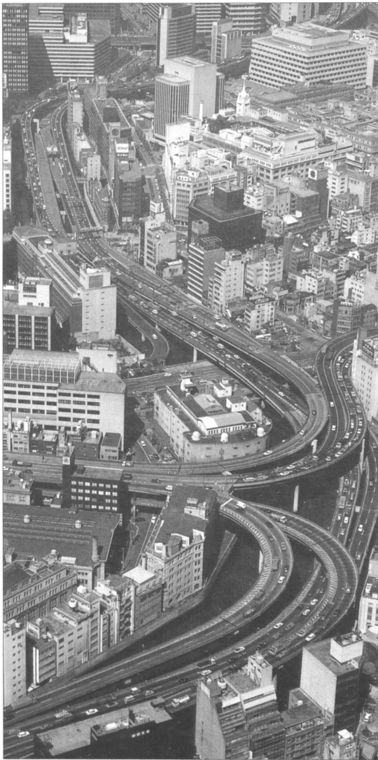
Figure 3.1 A portion of the Metropolitan Expressway illustrating routing over rivers and canals to minimize the disruption of property and to avoid the incredible costs of Japanese real estate.
