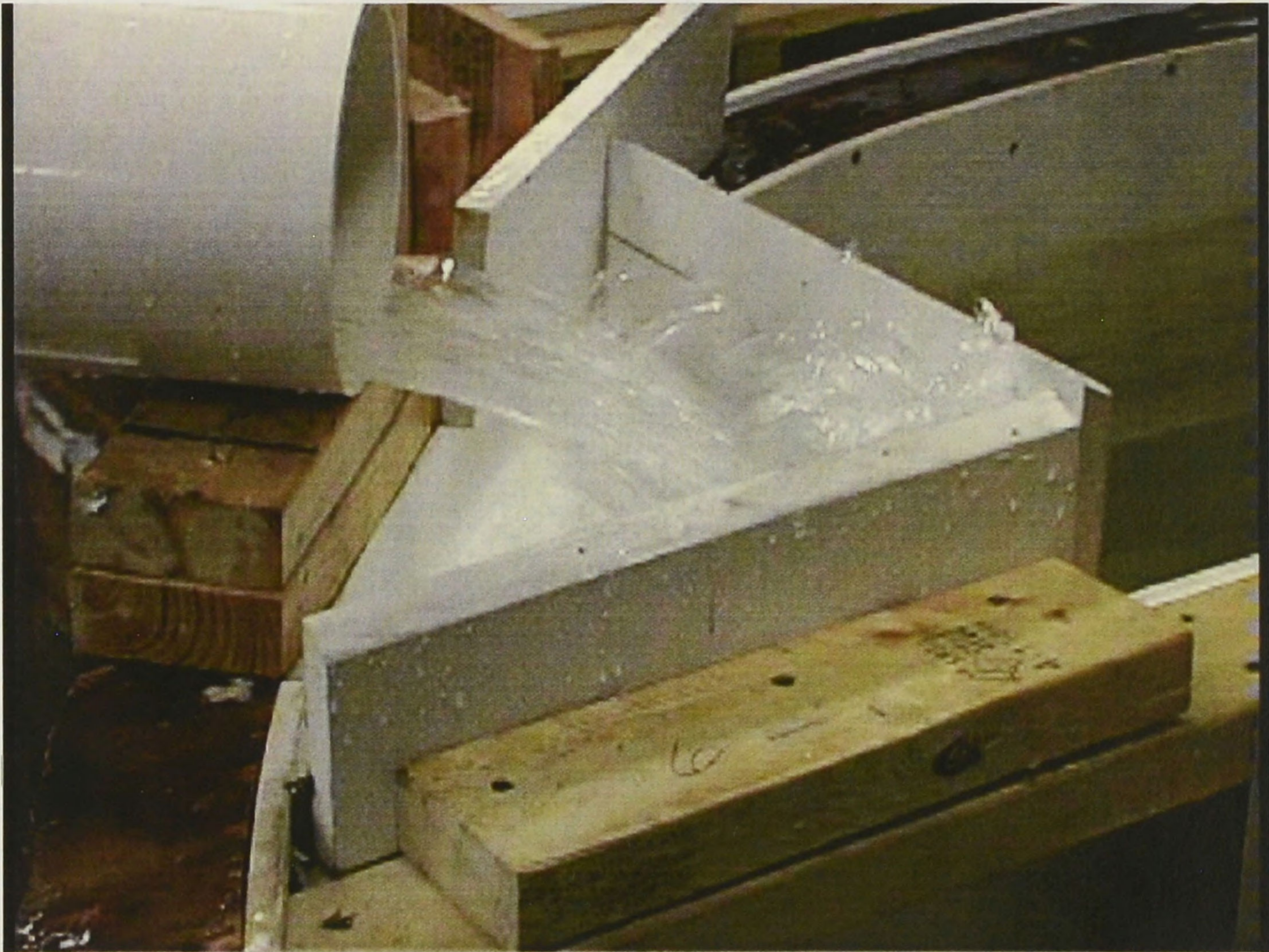
Figure 17. Detail of the discharge of the recycle flow into the wet well.
