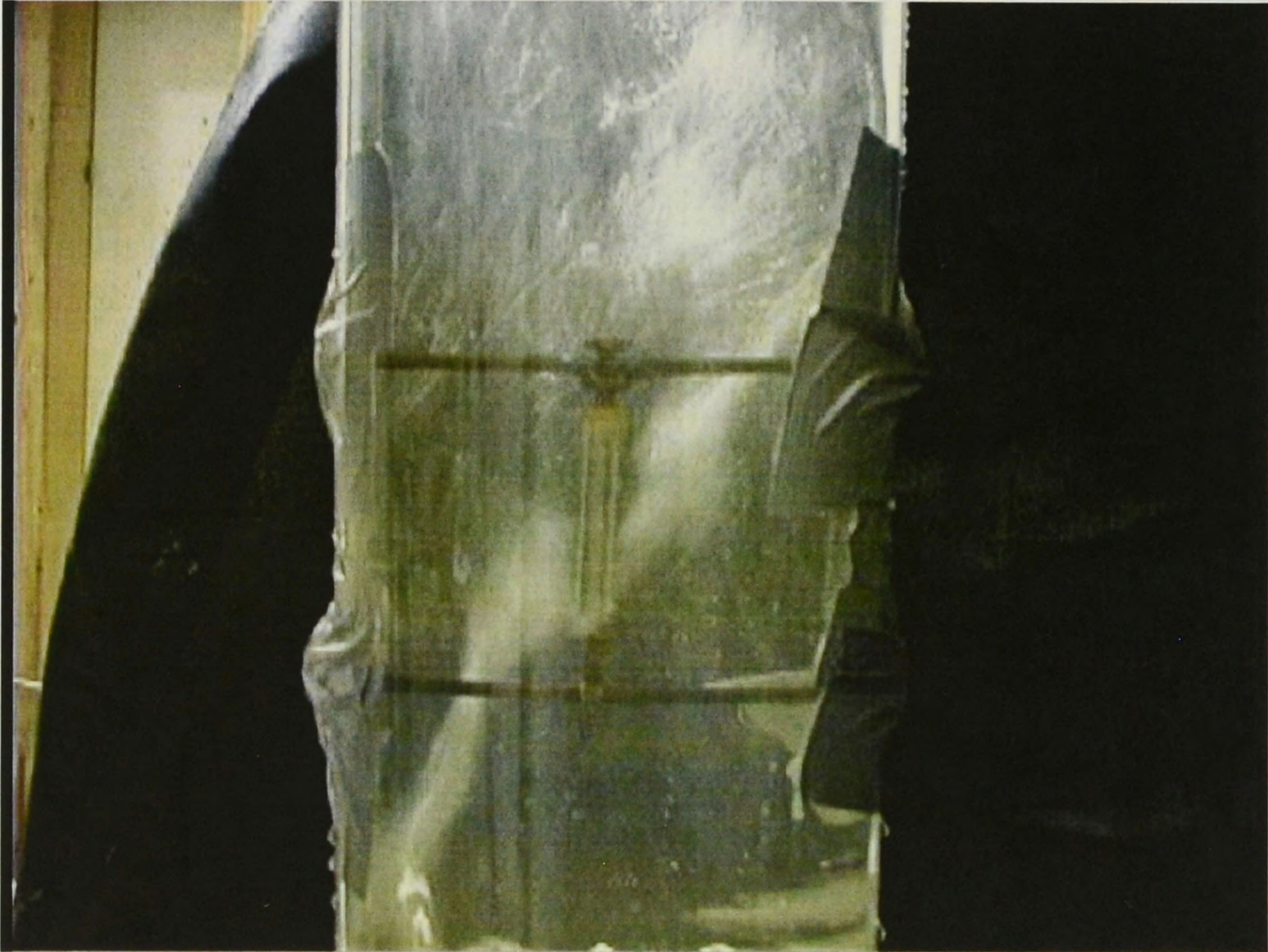
Figure 10. An air-entraining vortex into Pump #5.
