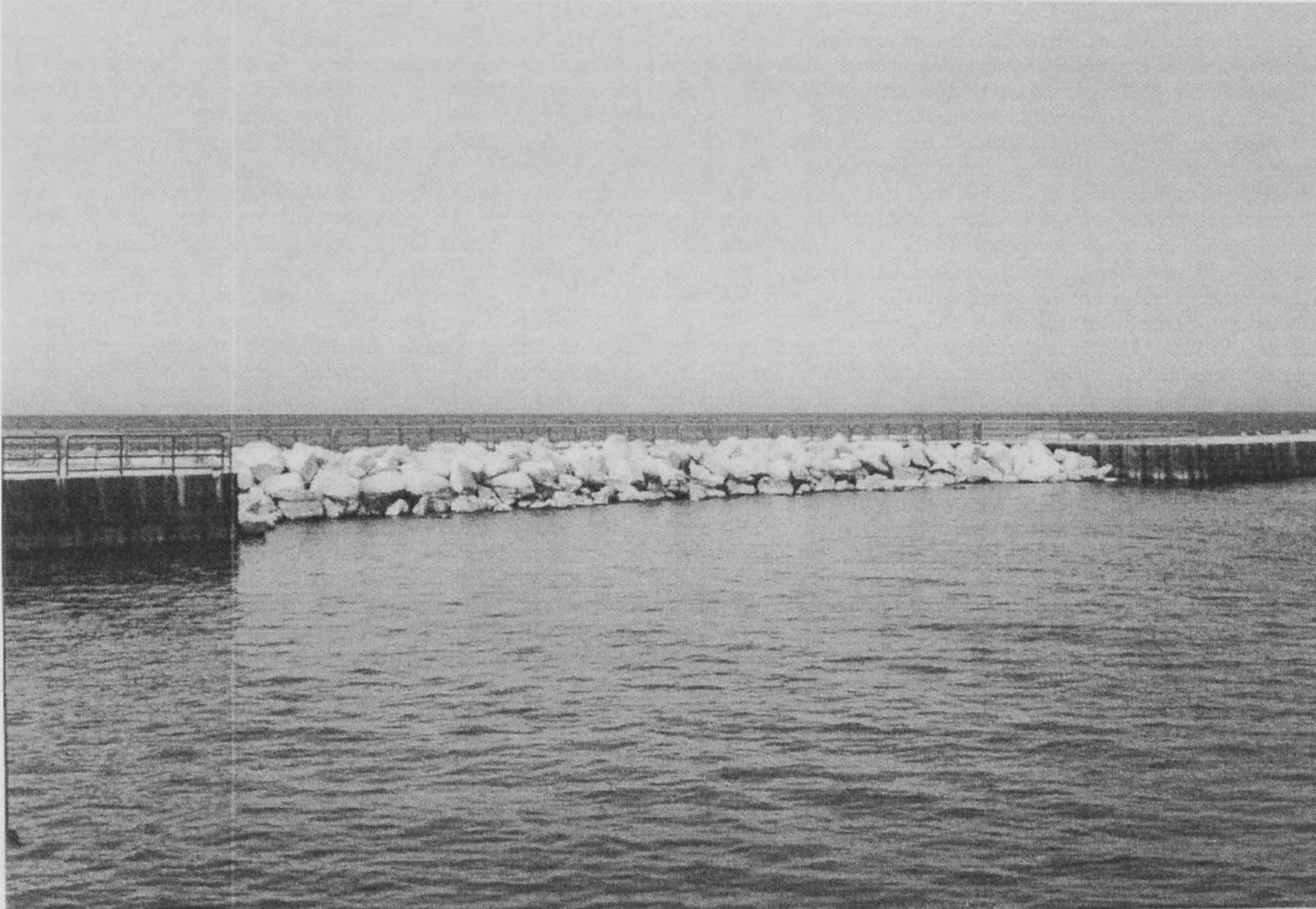
Figure 2: South pocket wave absorber at Pentwater, MI.
