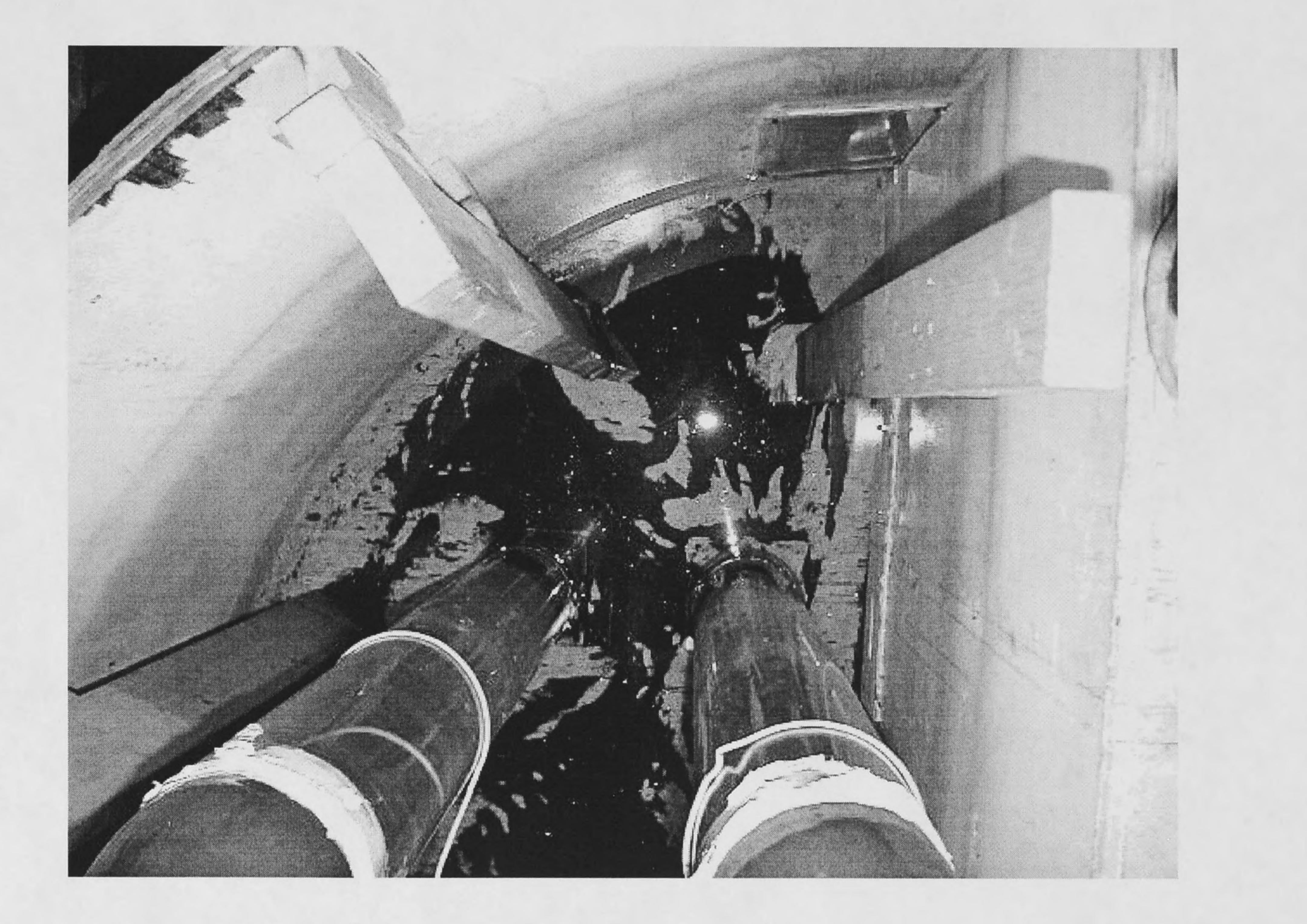
Figure 15. Sedimentation Patterns Behind Intakes 2 and 3.
