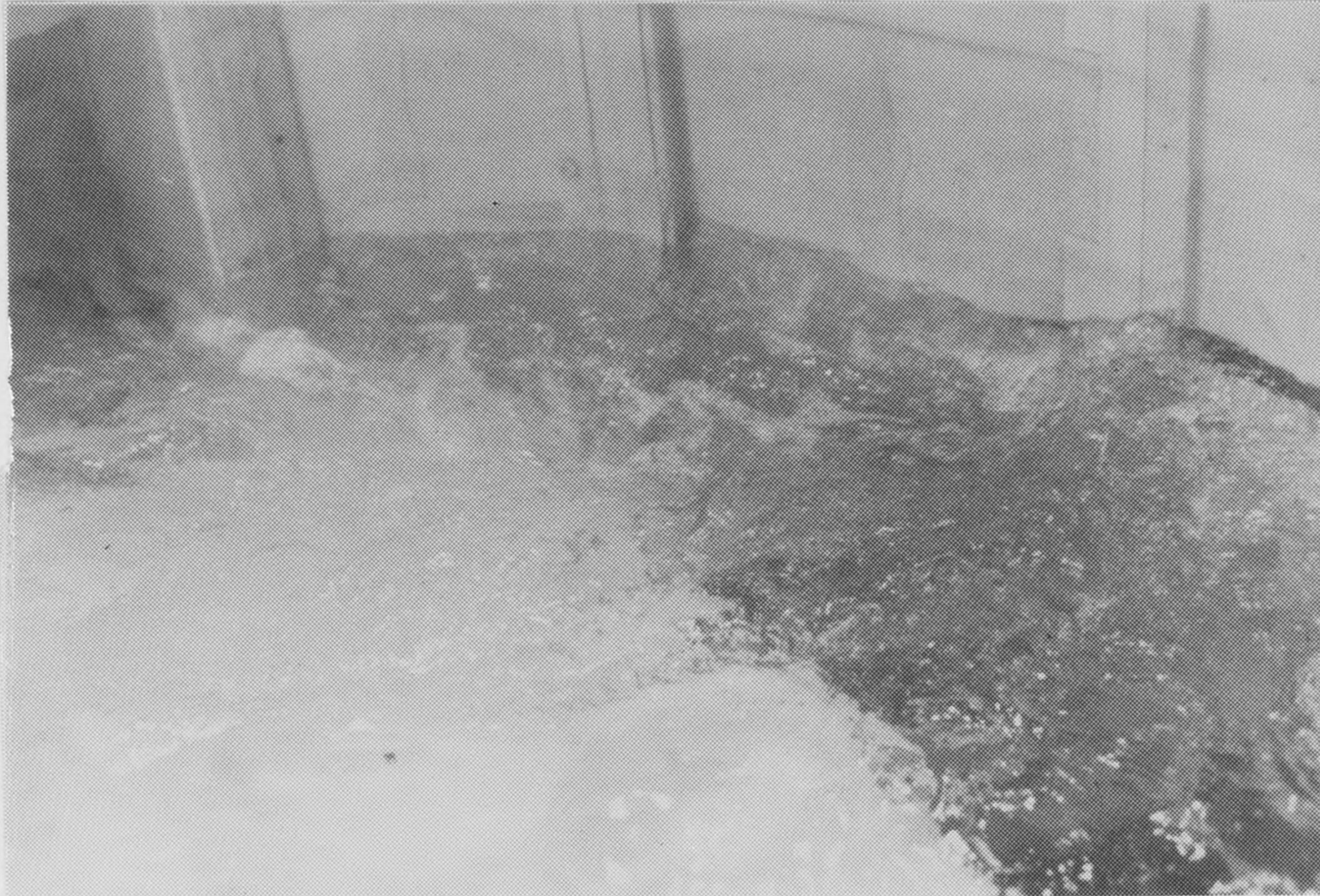
c.) View Inside of Wet Well from Center Dividing Wall.
