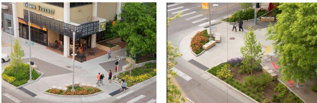
Figure 17. Bird's-eye view of the series of rain gardens that build on the planting strip
