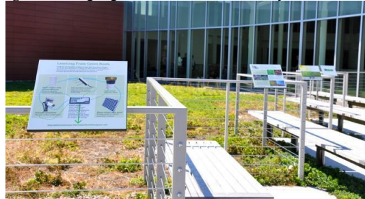
Figure 27. HUB Green roof signage
