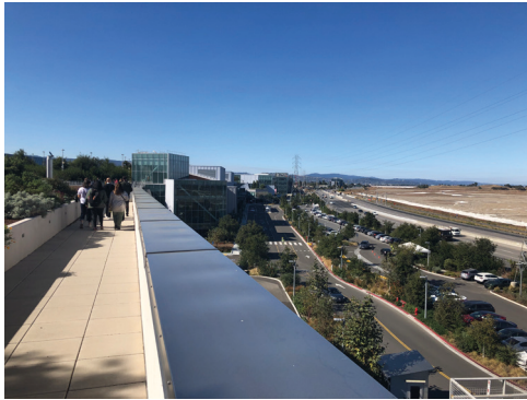
Figure 9. MPK rooftop and Menlo Park Salt Flats (Falkowski, 2019).
