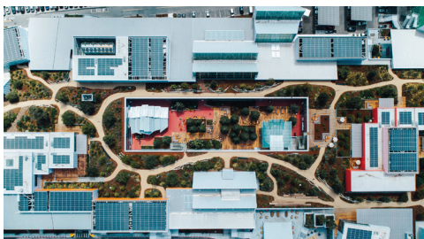
Figure 2. View of MPK 21 rooftop (Eleanor Gibson, Dezeen, 2018).
