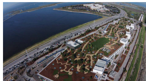
Figure 3. Aerial view of Facebook campus (Paul Moran, Level 10 Construction).
