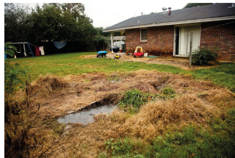
Figure 2. A home with a failing septic system in Lowndes County, Alabama (Anna Leah, Huffington Post, 2018).
