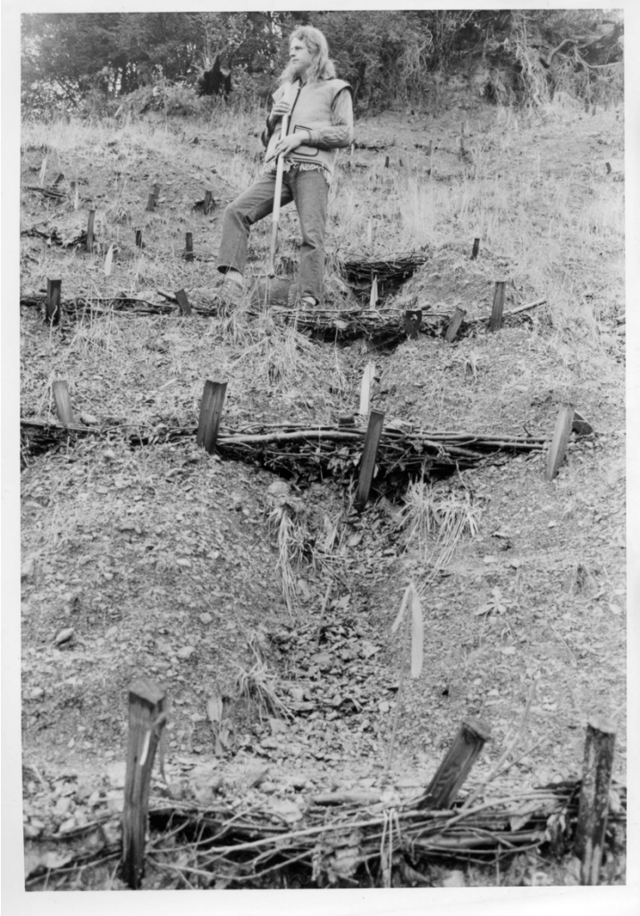
Figure 36 Early Park Service effort to address erosion following a landslide in Berry Glenn (National Park Service 2018d)
