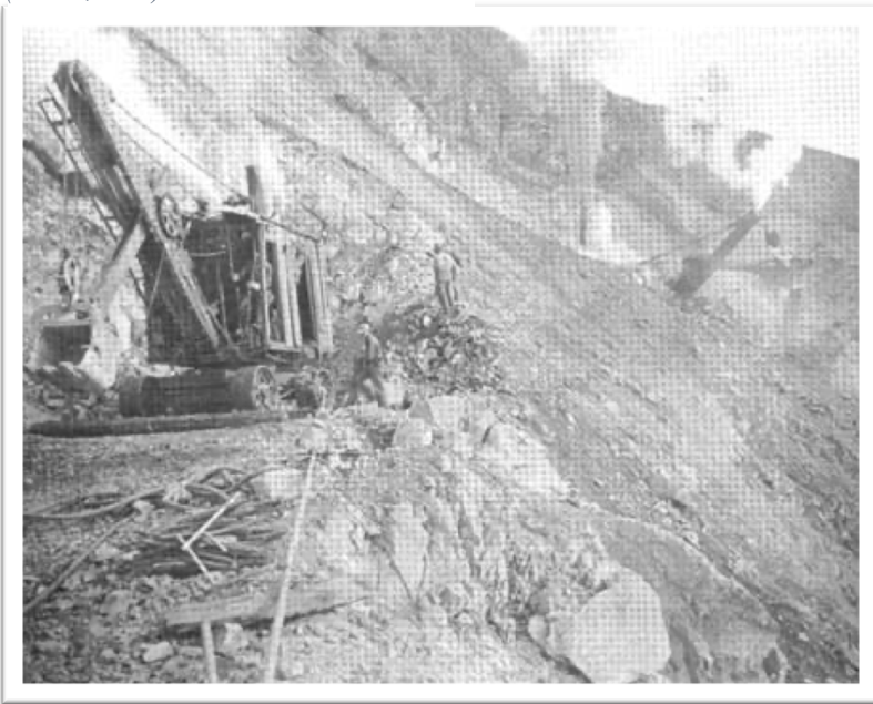
Figure 14 Construction of the Redwood Highway along the Cliffs South of Cushing Creek, Del Norte County, CA 1922 (Bearss 1969)
