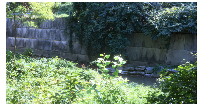
Top: Flooding in the Washington, D.C. Cleveland Park Metro station shut down the station and inconvenienced many.
