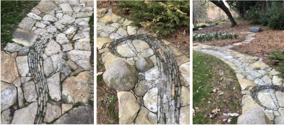
Figure-16. Drainage channel patterns. Photo by Zibo Zhu. 2019
