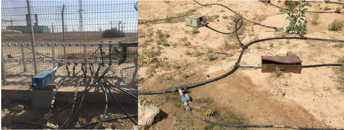
Figure 4.2. Examples of drinking water access for the Negev Bedouin: (left) “private” standpipe allowing connections to the public water source; (right) plastic tubes transporting water from a public source to Bedouin households; both photographs taken by Grace Christensen, Emory University
