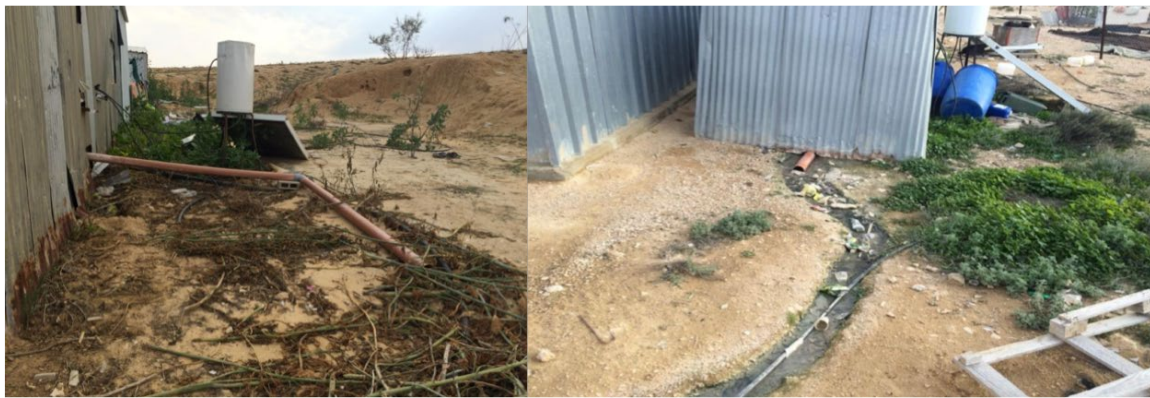
Figure 4.3. Examples of sanitation facilities for the Negev Bedouin: two examples of sanitation facilities transmitting sewage directly into the environment
