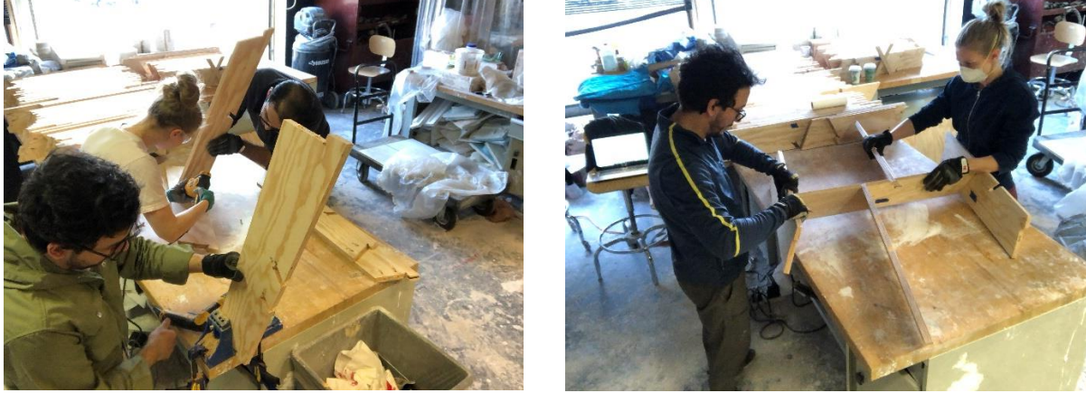
Figure 222_ Predrilling the screws and pre-assembly of connecting members.
