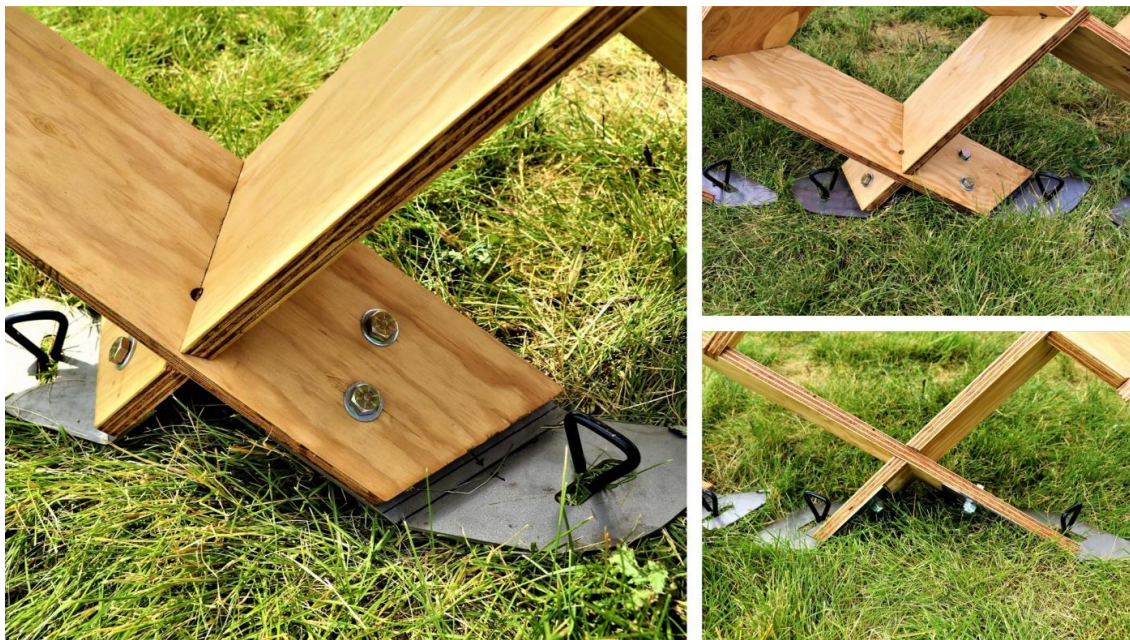
Figure 233_ Base plate connection detailing.
