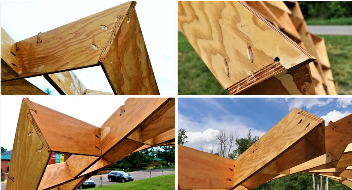
Figure 237_ Arch connection detailing.
