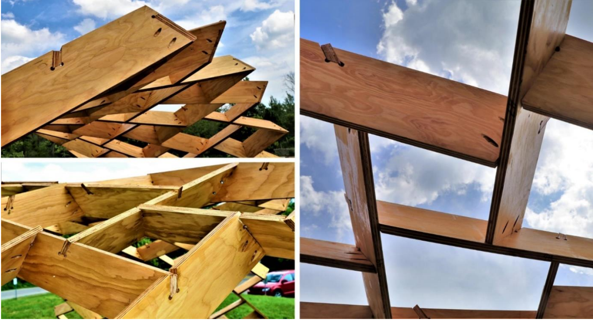
Figure 236_ Arch connection detailing.
