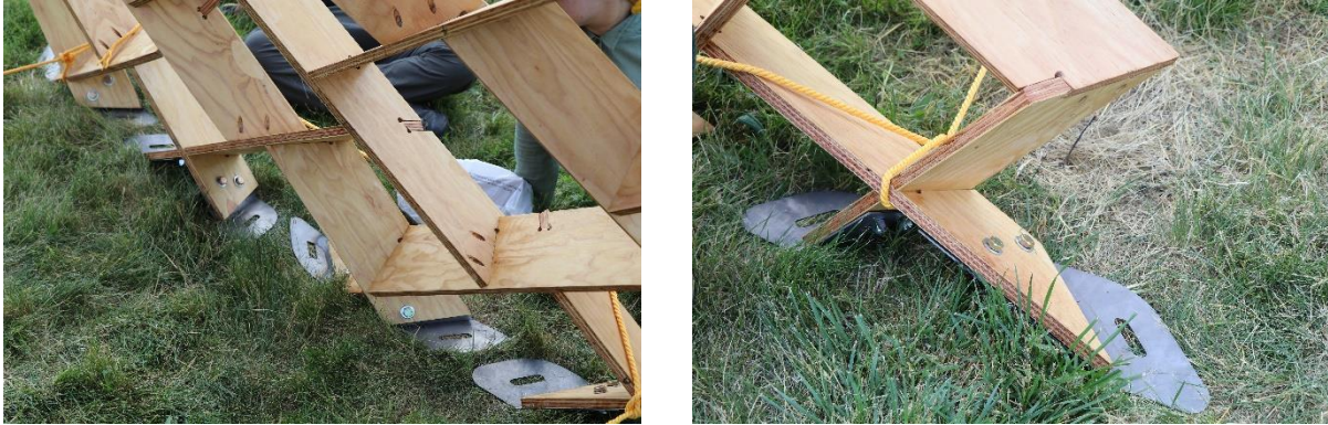
Figure 232_ Connecting the base plates to the arch support members.
