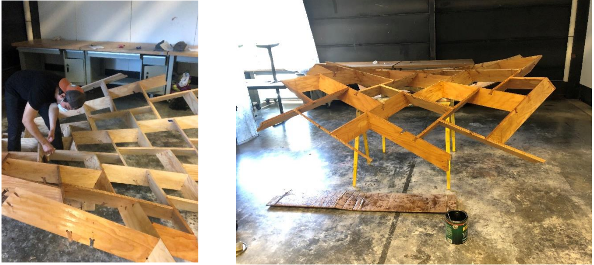
Figure 224_ Application of waterproof and anti UV sealant to the arch.
