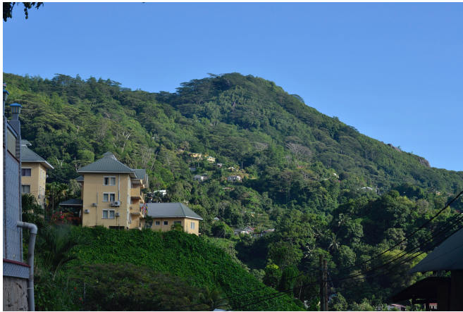
Photo 2.6. Structures built into the steep incline of the central mountainous peak on Mahé.
