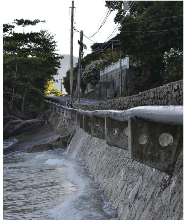
A utility line runs along a coastal road in Bel Ombré.
