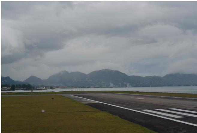
Photo 2.1. Runway at Seychelles International Airport adjacent to the ocean.
