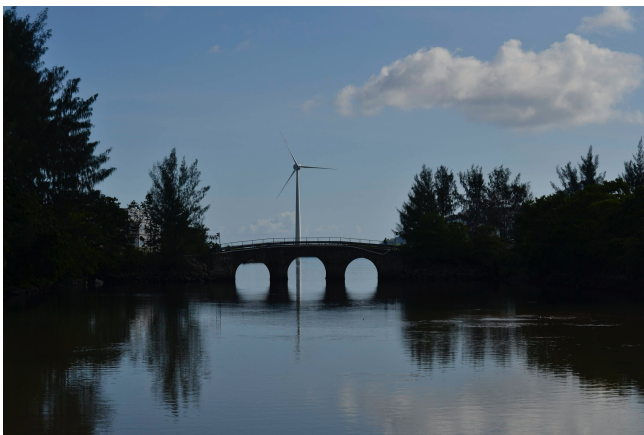
Photo 1.6. Off-shore wind turbine seen from East Coast Road in Victoria.
