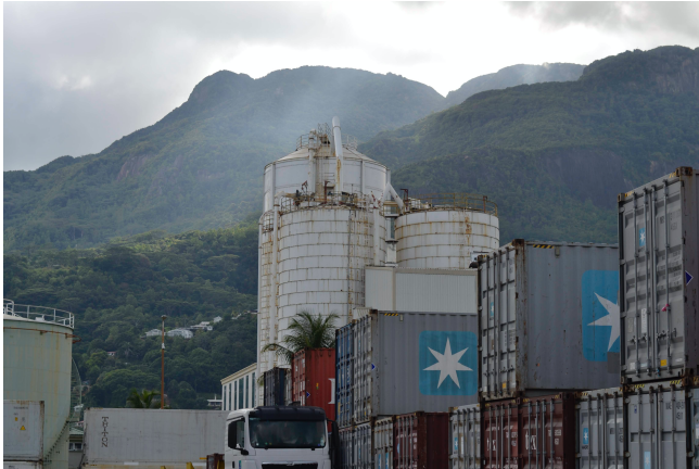
Photo 1.5. Silos storing oil at the Seychelles Petroleum Depot in Victoria.
