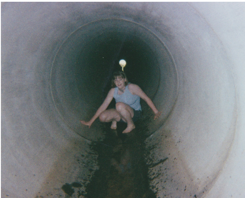
Fig. 3. Snapshot of me in a stormwater culvert
