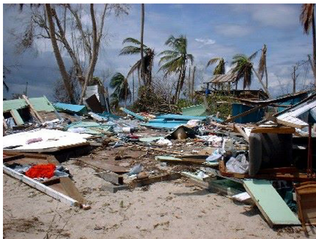
FIGURE 2. Image of Placencia Village post Hurricane Iris, 2001.
