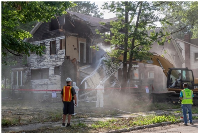
Figure 20 A news image of an emergency demolition captioned, “Dust envelops a worksite as workers, using protective clothing to guard against asbestos exposure demolish an abandoned house.” Observers include a regulatory worker and supervisor from the Detroit Building Authority. Photo by Jim West. Rights Acquired.
