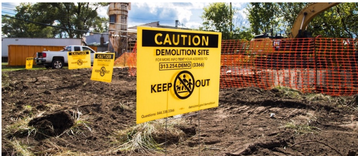
Figure 3 Demolition in progress. Image from City of Detroit digital archive
