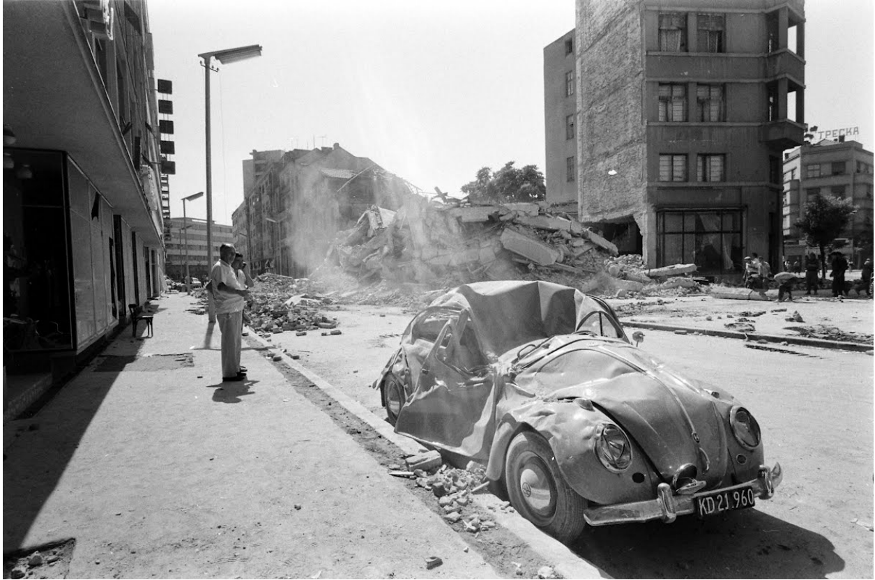
Figure 26: 26 July 1963 earthquake. Skopje, Macedonia. Immediate aftermath.
