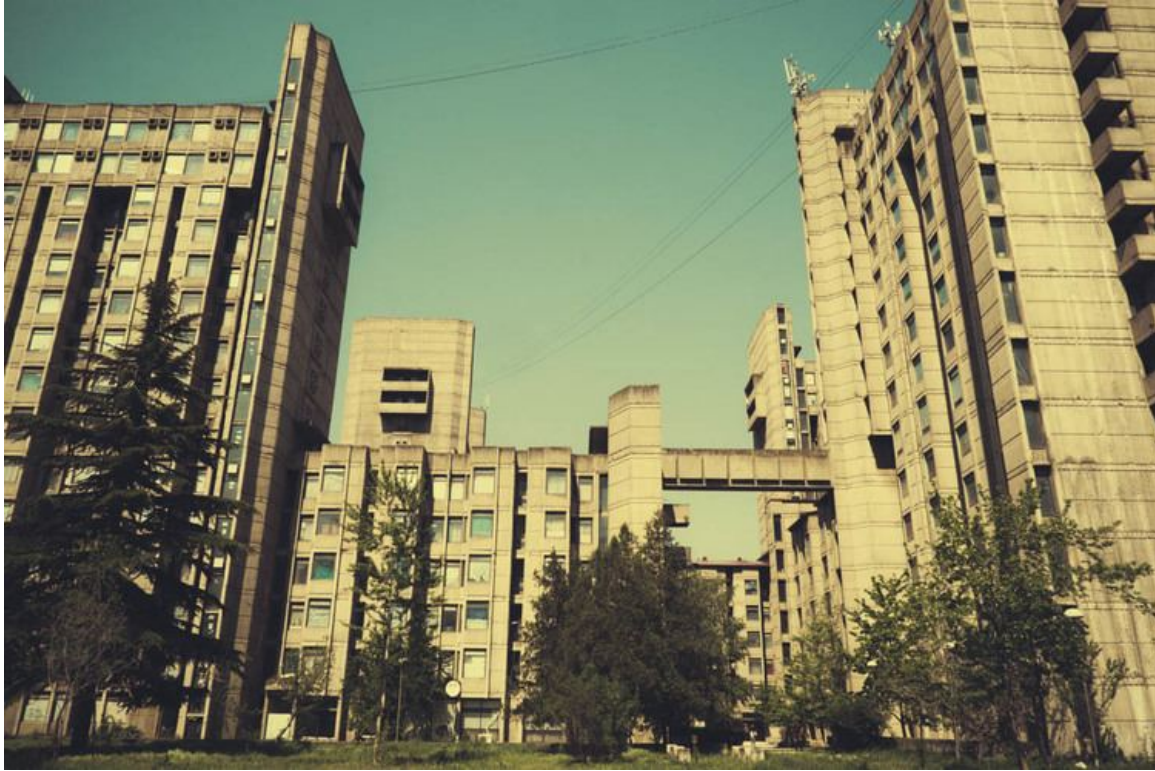
Figure 62: Goce Delčev Student Dormitories. Skopje, Macedonia. 1969-1971 and 1973-1977. Architect: Georgi Konstantinovski.
