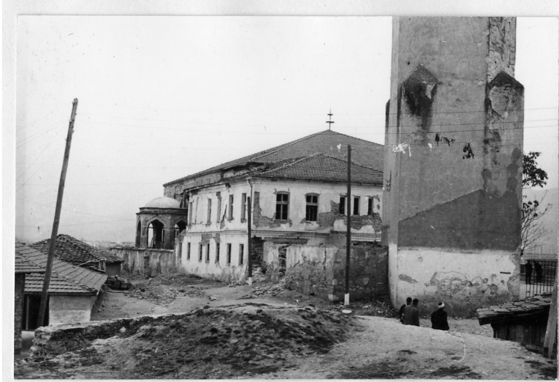
Figure 76: Ottoman Old Town. 1963 earthquake destruction. Skopje, Macedonia.
