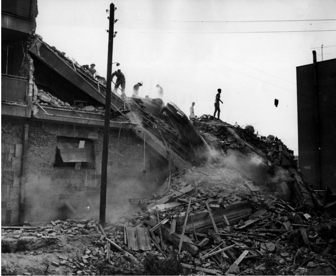
Figure 33: Destruction of Skopje earthquake and clearing of rubble. Skopje, Macedonia.
