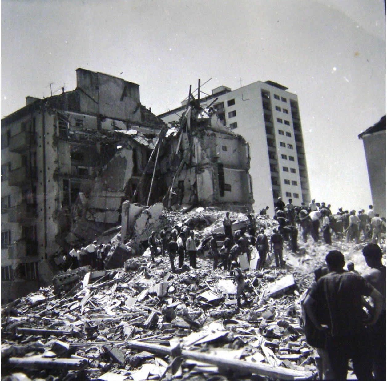
Figure 30: Clearing the rubble. Post-earthquake. Skopje, Macedonia.
