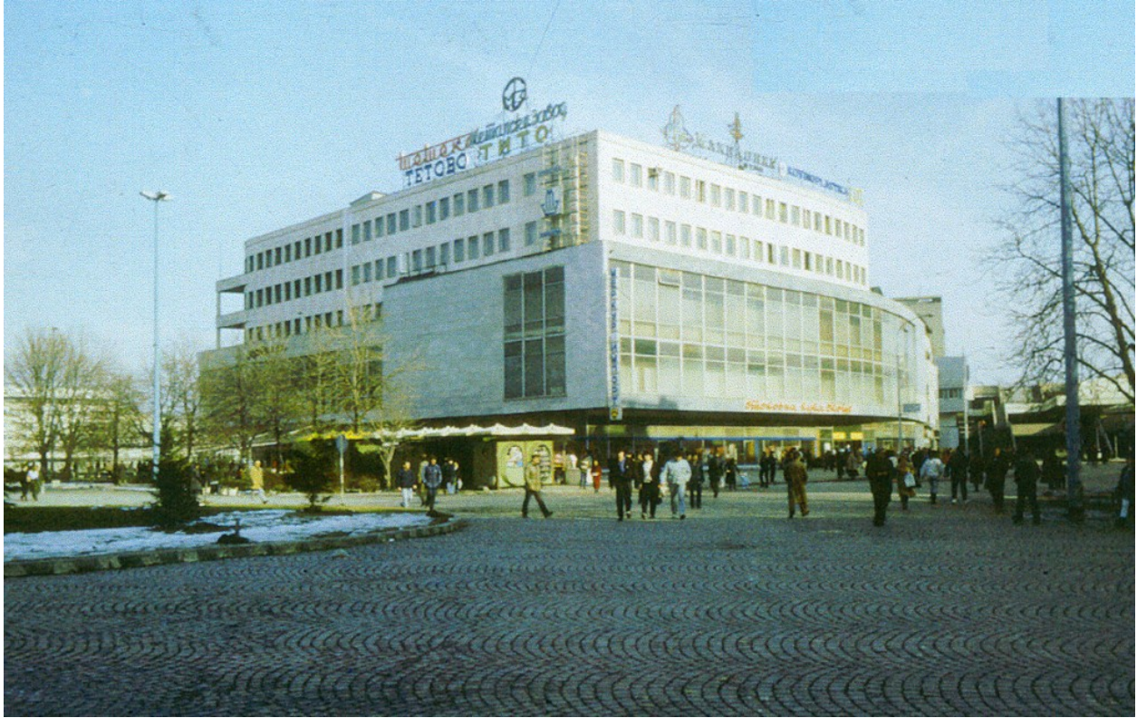
Figure 18: NAMA department store. Skopje, Macedonia. 1959. Architect: Slavko Brezovski.
