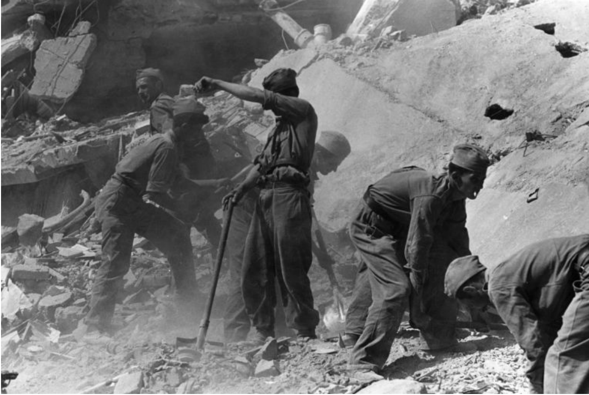
Figure 32: Destruction of Skopje earthquake and clearing of rubble. Skopje, Macedonia.
