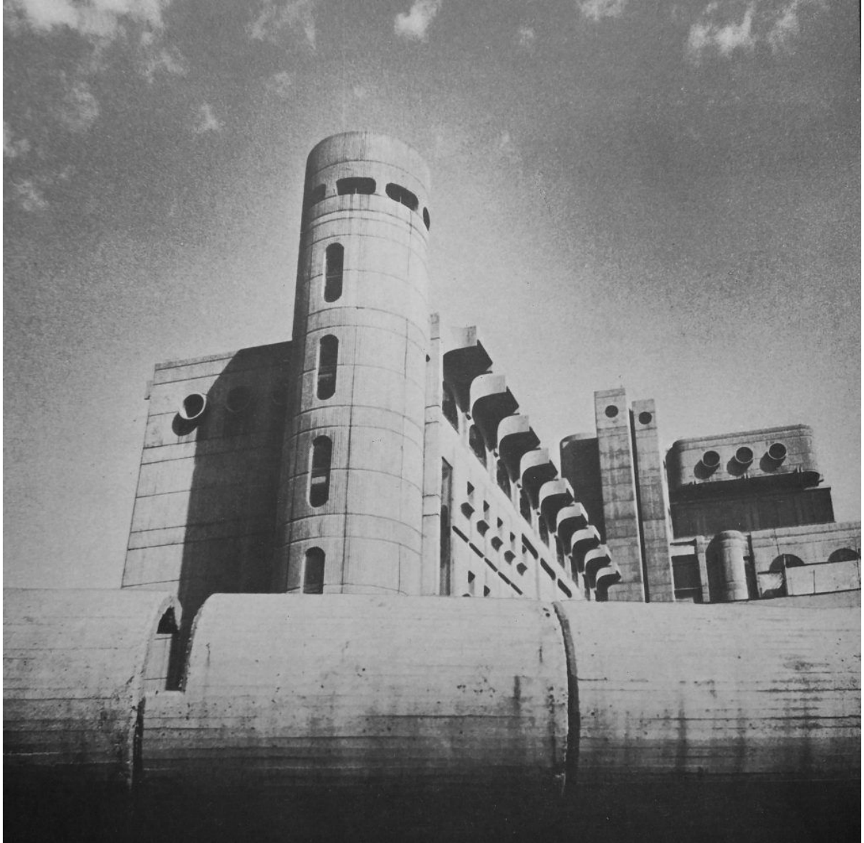
Figure 72: Telecommunications Center. Detail. Skopje, Macedonia. 1979-1981. Architect: Janko Konstantinov.
