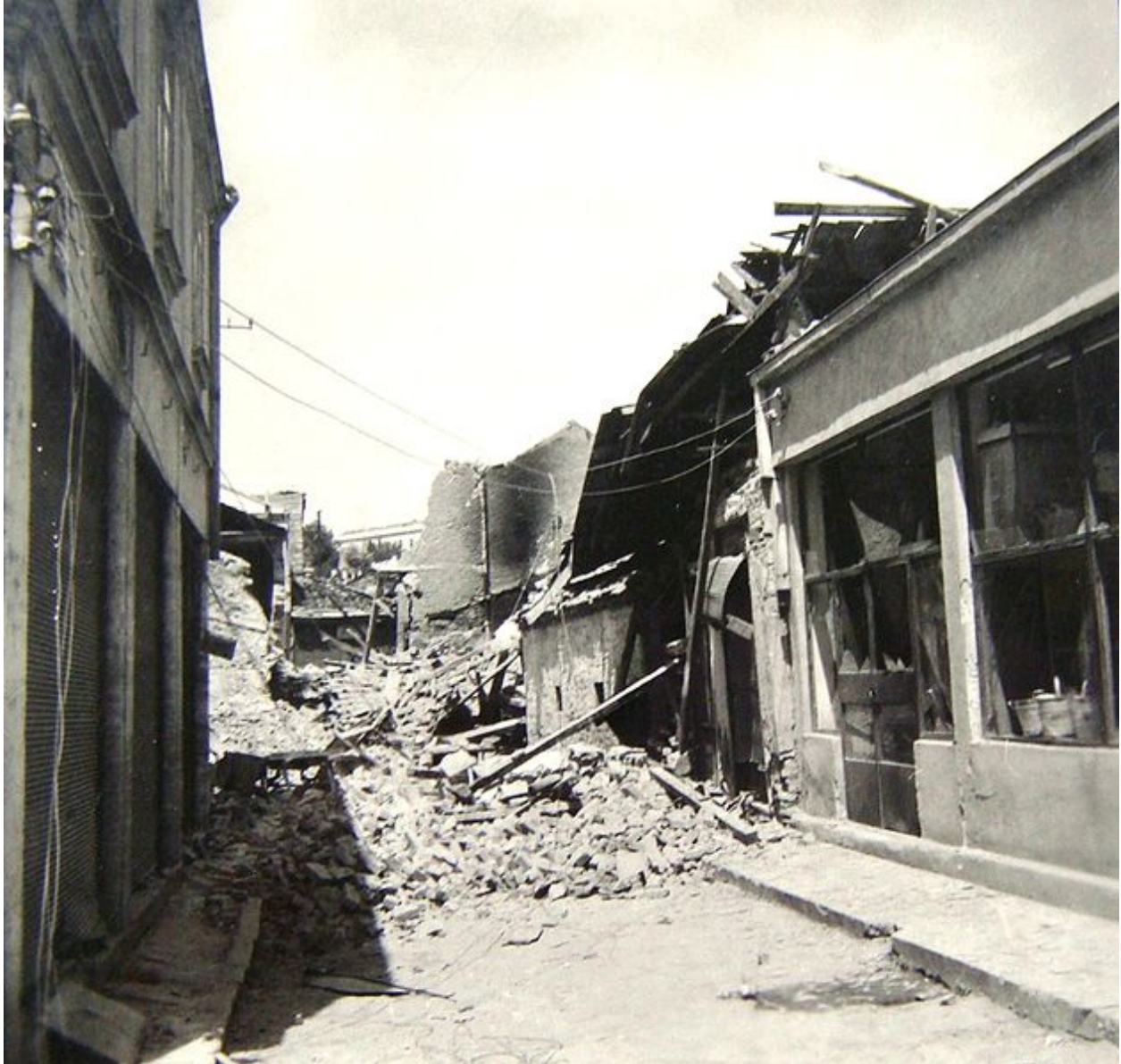
Figure 79: Ottoman Old Town. 1963 earthquake destruction. Skopje, Macedonia.
