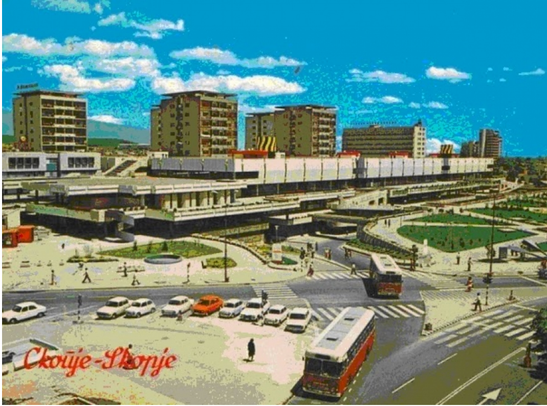
Figure 66: GTC shopping center. Skopje, Macedonia. 1969-1973. Architect: Živko Popovski.
