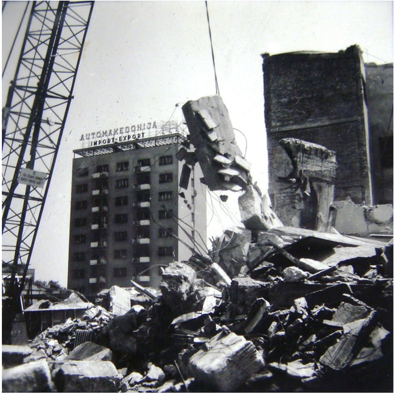
Figure 35: Destruction of Skopje earthquake and clearing of rubble. Skopje, Macedonia.
