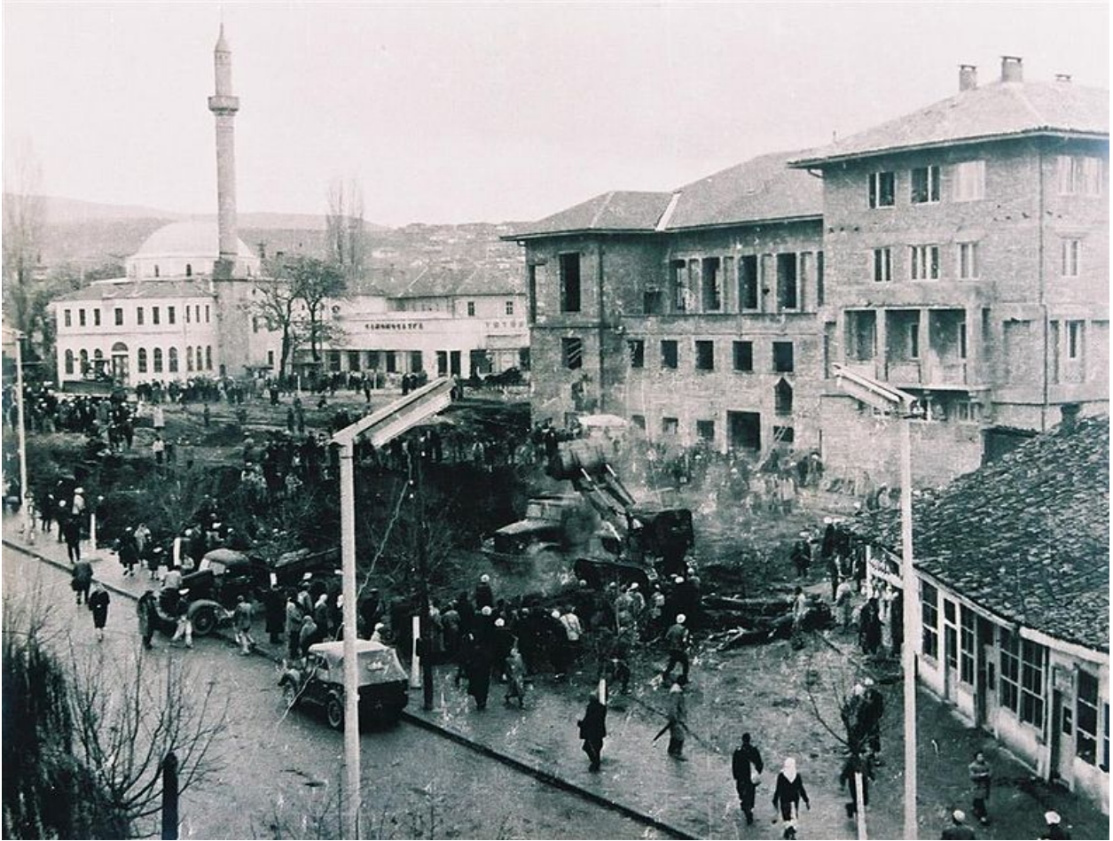
Figure 21: Demolition of Pridstina Ottoman Bazaar. Postwar. Pridstina, Kosovo.
