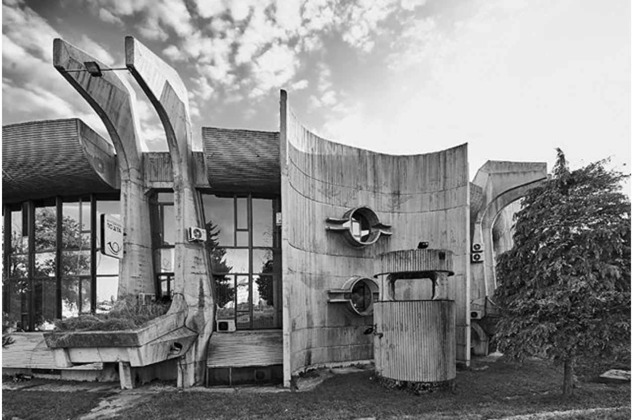
Figure 73: Telecommunications Center. Detail. Skopje, Macedonia. 1979-1981. Architect: Janko Konstantinov.
