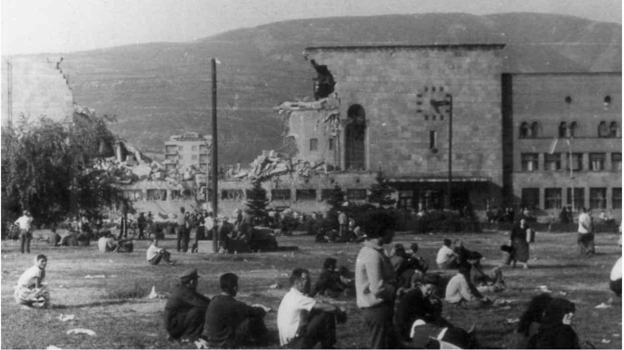
Figure 25: 26 July 1963 earthquake. Railway Station. Skopje, Macedonia. Immediate aftermath.
