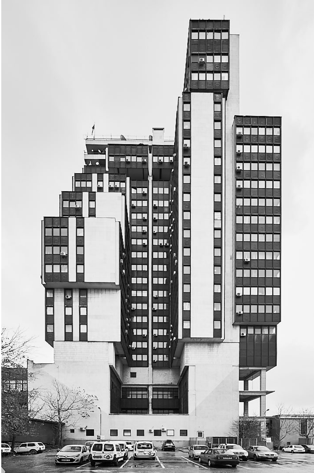
Figure 74: Macedonian Radio and Television Center (MRT). Skopje, Macedonia. 1973-1984. Architects: Kiril Acevski, Nakov Manov, and Haralampsi Josifovski.
