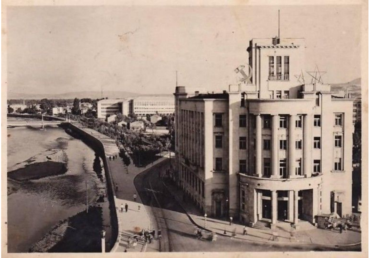
Figure 7: National Bank. Skopje, Macedonia. 1931. Architect: Bogdan Nestorović.
