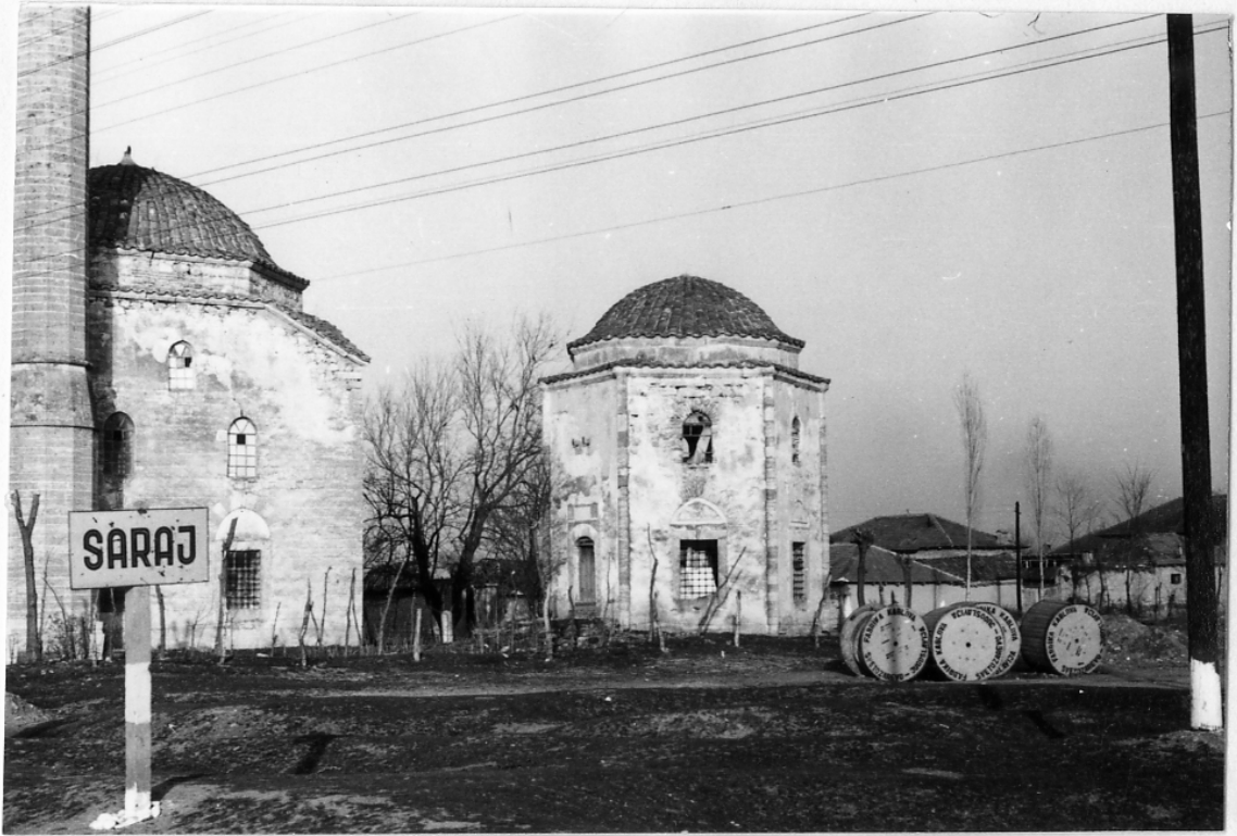
Figure 77: Ottoman Old Town. 1963 earthquake destruction. Skopje, Macedonia.
