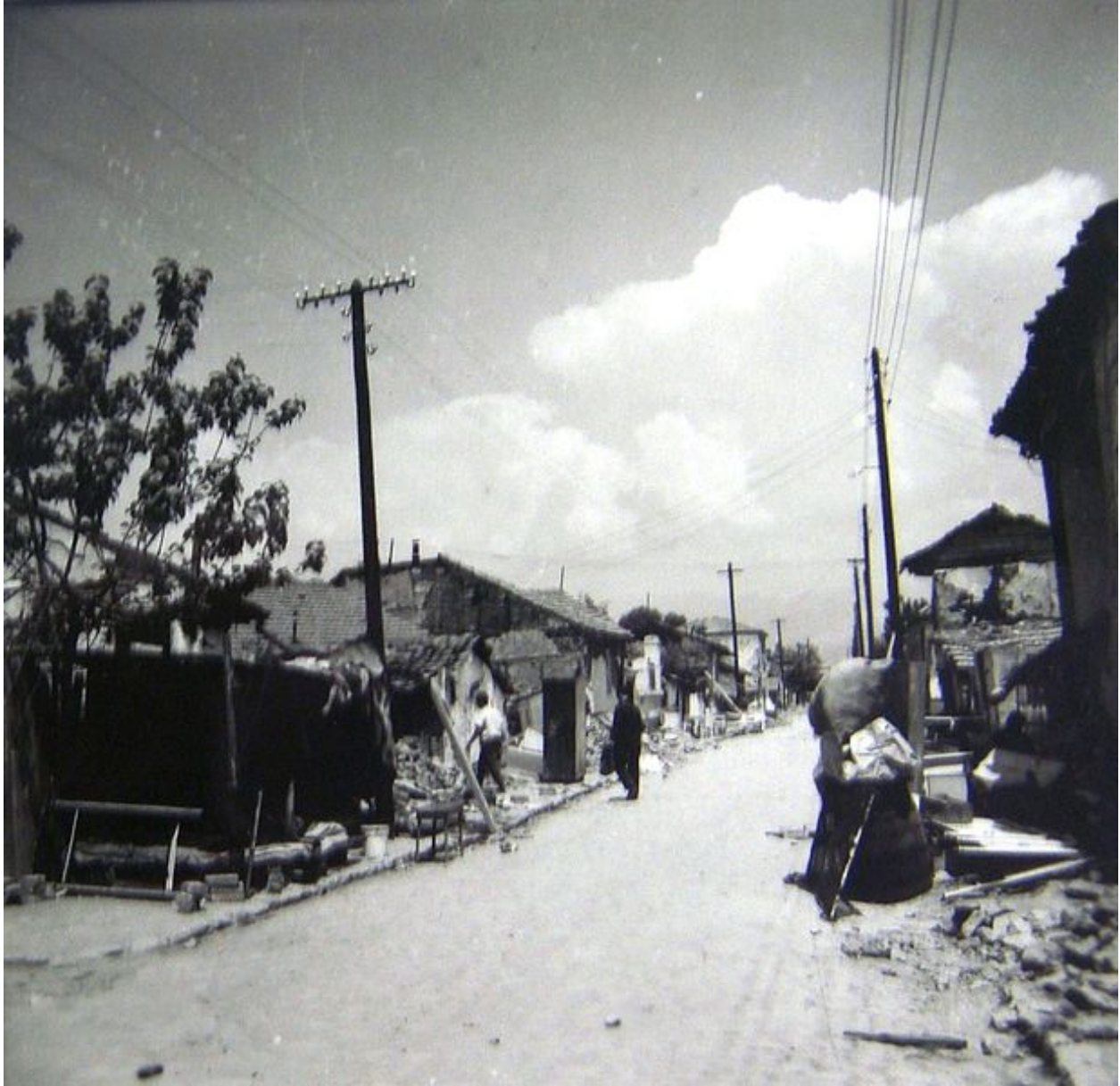
Figure 78: Ottoman Old Town. 1963 earthquake destruction. Skopje, Macedonia.
