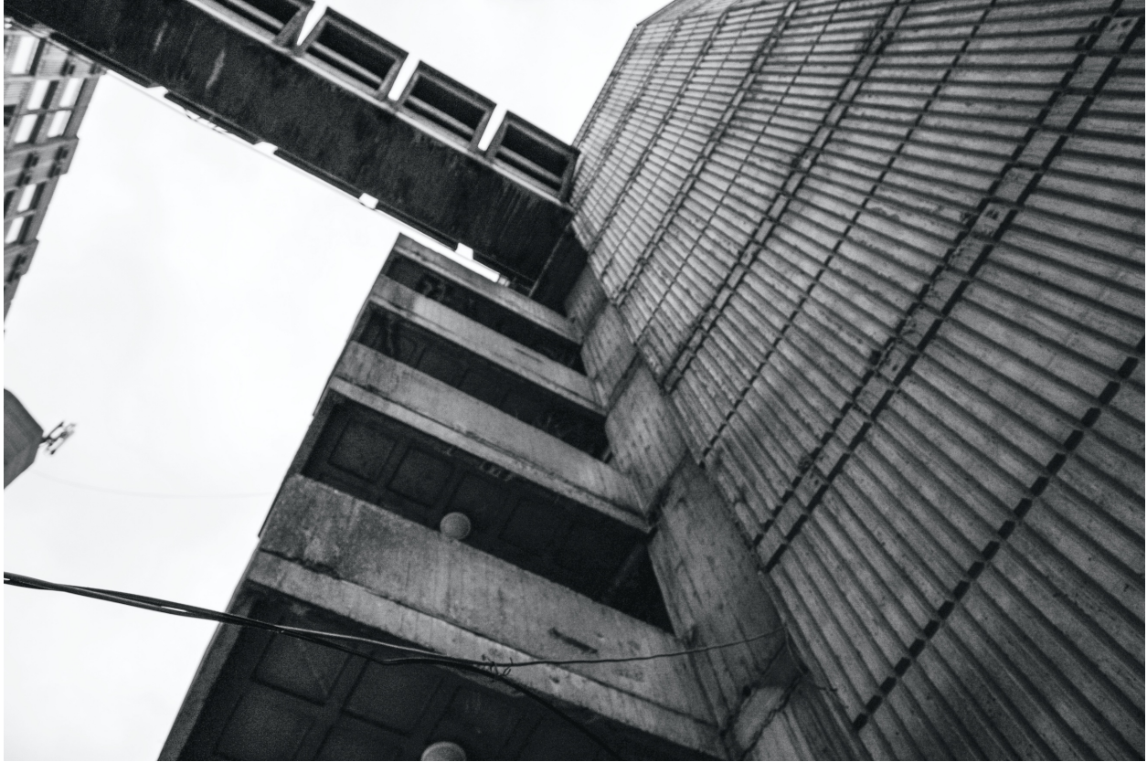
Figure 63: Goce Delčev Student Dormitories. "Flying bridges." Skopje, Macedonia. 1969-1971 and 1973-1977. Architect: Georgi Konstantinovski.
