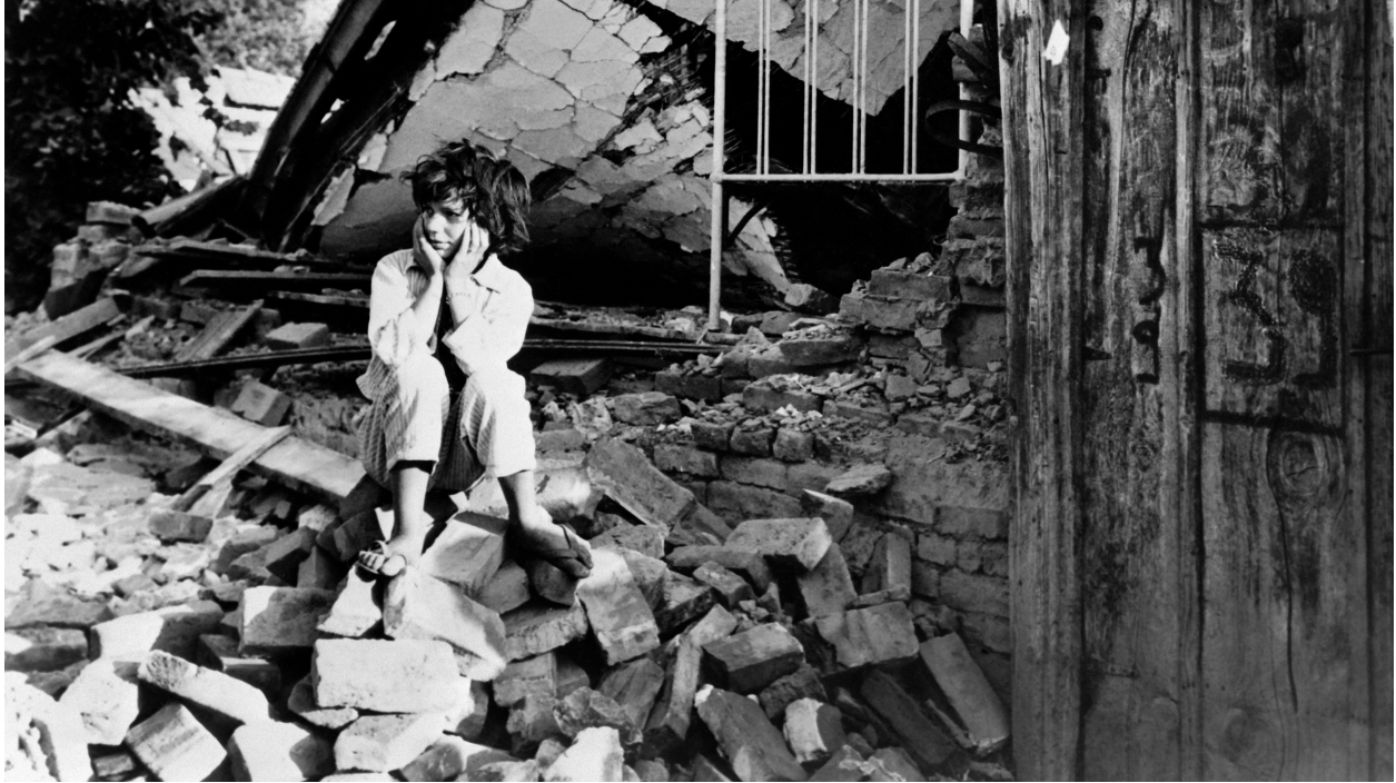
Figure 31: Destruction of Skopje earthquake. Skopje, Macedonia.
