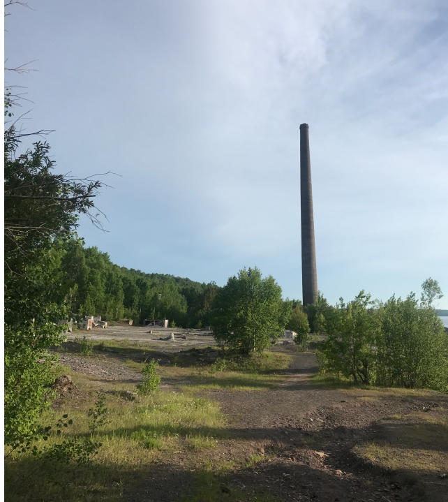
Figure 3.2: The remnants of the Champion Copper Mill in Freda, Michigan. Abandoned mining infrastructure is widespread through the Keweenaw Peninsula. Photo by author.
