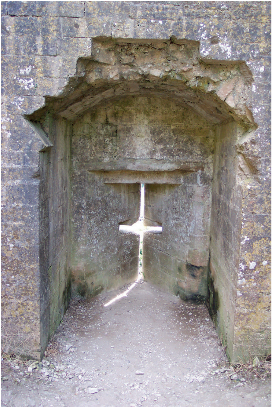
FIGURE 2.5 Interior perspective of loop-hole at Corfe Castle, Dorset, England. Source: John Bointon, under Creative Commons License Attribution 2.0 Generic (CC BY 2.0).
