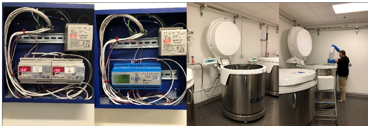
Figure 1: Old gas detection system. Issues with faulty oxygen sensor revealed inability to record oxygen levels in Biorepository. Connection to UM BAS only allowed 30 minute interval recording.
