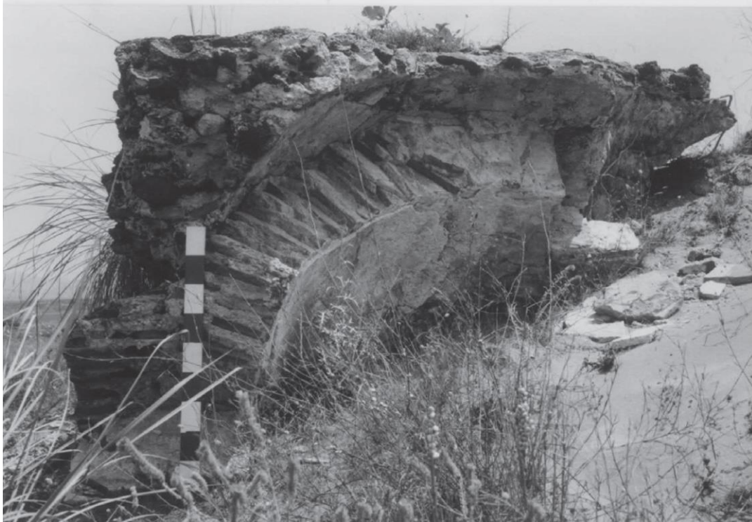
Figure 153: Close-up view in the Smaller Baths at Küçük Bernaz, showing radially set bricks in the intrados of Room C and mortared rubble packing above it (Tobin 2004, fig. 42).
