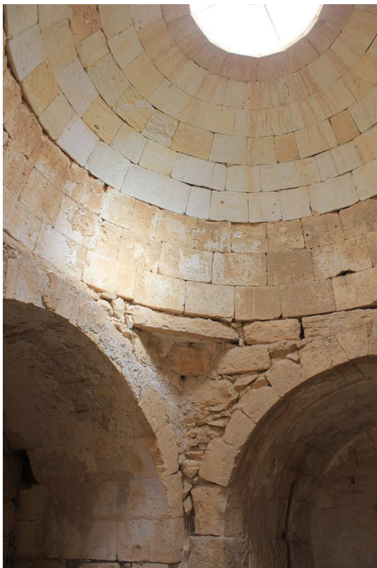
Figure 177: Interior view of the caldarium of the baths at Oboda (modern Avdat), showing partially reconstructed ashlar dome resting on squinches formed by a single stone slab in the corners (photo by author).
