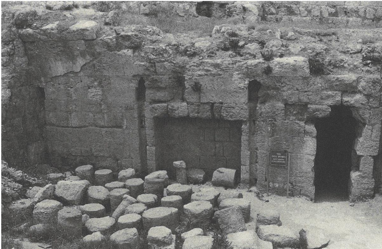
Figure 102: View of the caldarium of the upper baths at Herodium, showing ashlar masonry and the bottom courses of the ashlar vault on the left-hand side of the photo (Netzer 1999, fig. 7).
