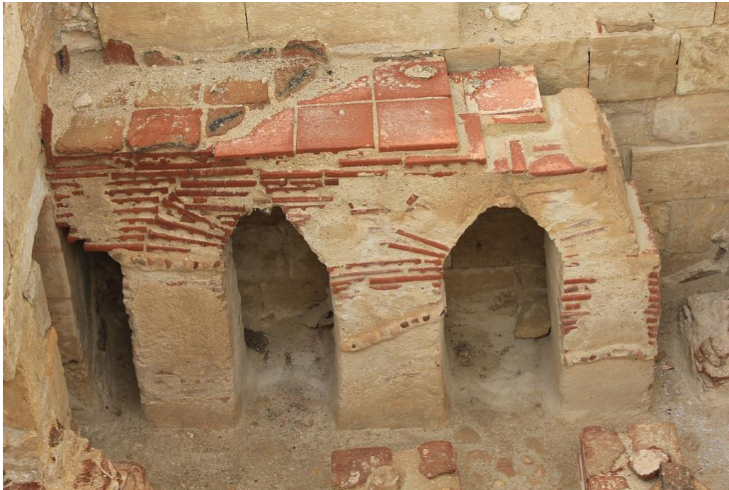
Figure 224: Reconstructed arched pilae in the hypocaust of the baths at Mamshit (Mamphis) (photo by author).
