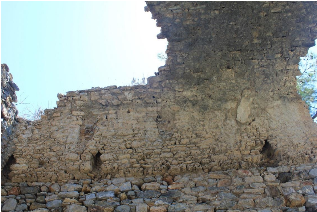
Figure 14: Interior of baths (“Building 6”) at Iotape, facing south, showing masonry of rough-cut limestone and vaulting of lime-tufa above (photo by author).
