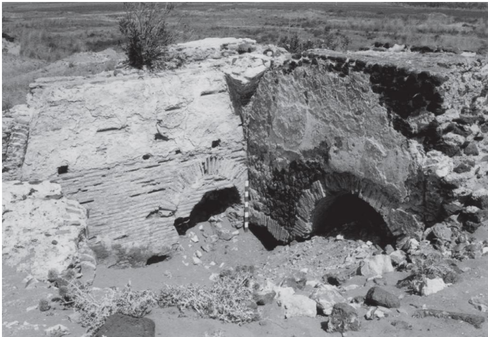
Figure 42: View of Room A of the Smaller Baths at Küçük Bernaz, showing mortared rubble walls faced brick and roughly shaped polygonal basalt stones (Tobin 2004, fig. 31).
