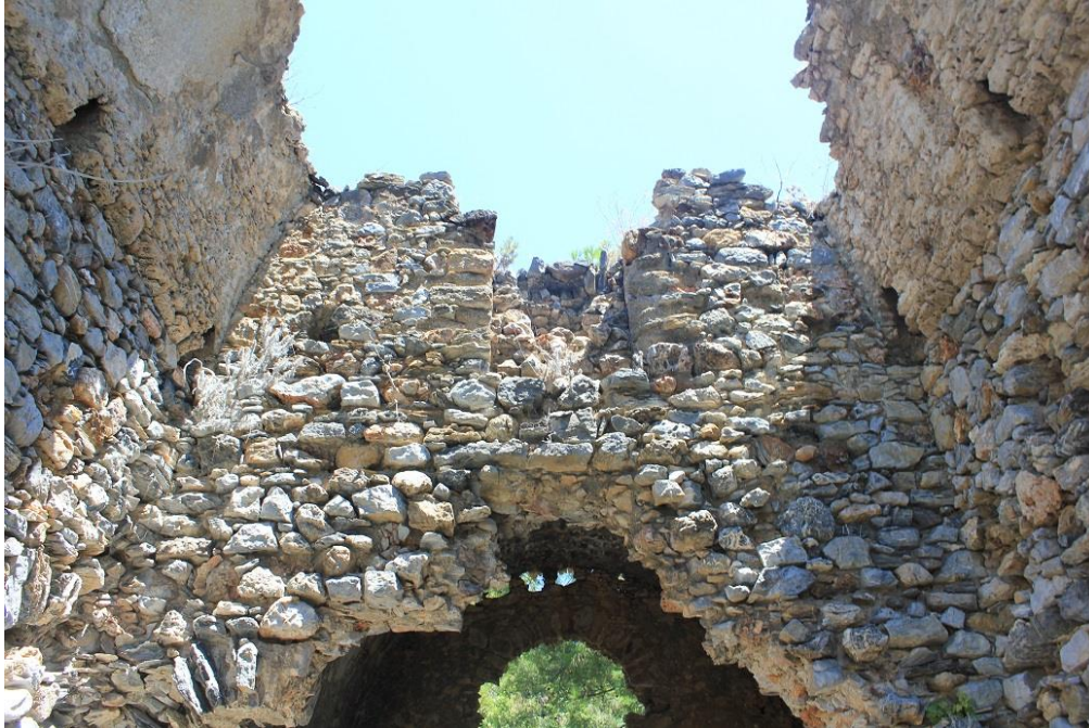
Figure 13: Interior of baths (“Building 6”) at Iotape, facing east, showing masonry of rough-cut limestone and vaulting of lime-tufa above (photo by author).
