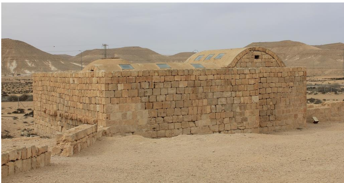
Figure 135: Exterior view of the baths at Oboda (modern Avdat), showing ashlar masonry (photo by author).
