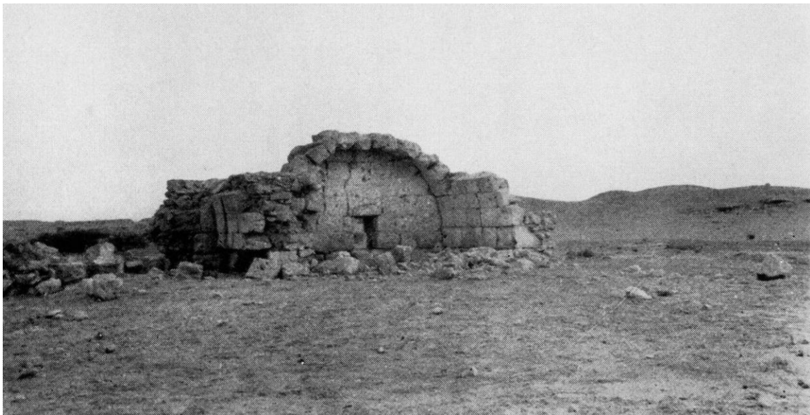
Figure 175: View of the baths at Tamara (modern En Hazeva), showing ashlar construction of the vaults (Glueck 1935, fig. 7).
