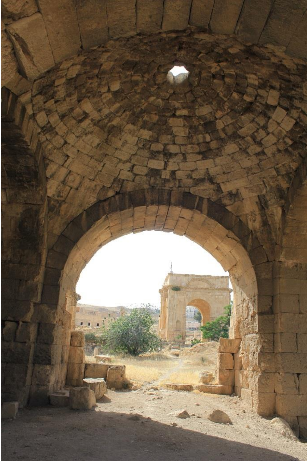
Figure 167: Interior view of the intact dome in the eastern hall of the West Baths at Gerasa (modern Jerash), showing the limestone ashlar construction of the dome and the use of pendentives to place a hemispherical dome over a square room (photo by author).
