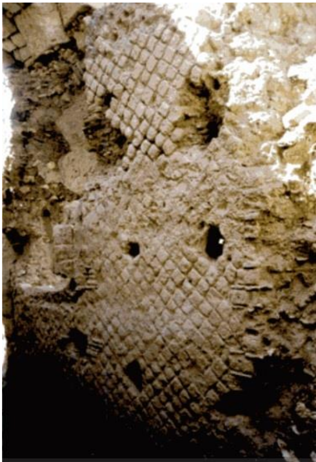
Figure 34: West wall of Room 12 in the Harbor Baths at Elaeussa Sebaste, showing use of opus reticulatum (Borgia and Spanu 2003, 237).
