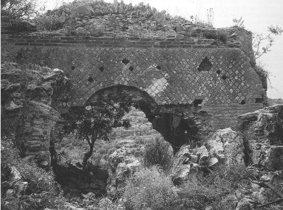
Figure 31: Exterior of Reticulate Baths at Elaeussa Sebaste, showing use of opus reticulatum (Spanu 1999, fig. 56).
