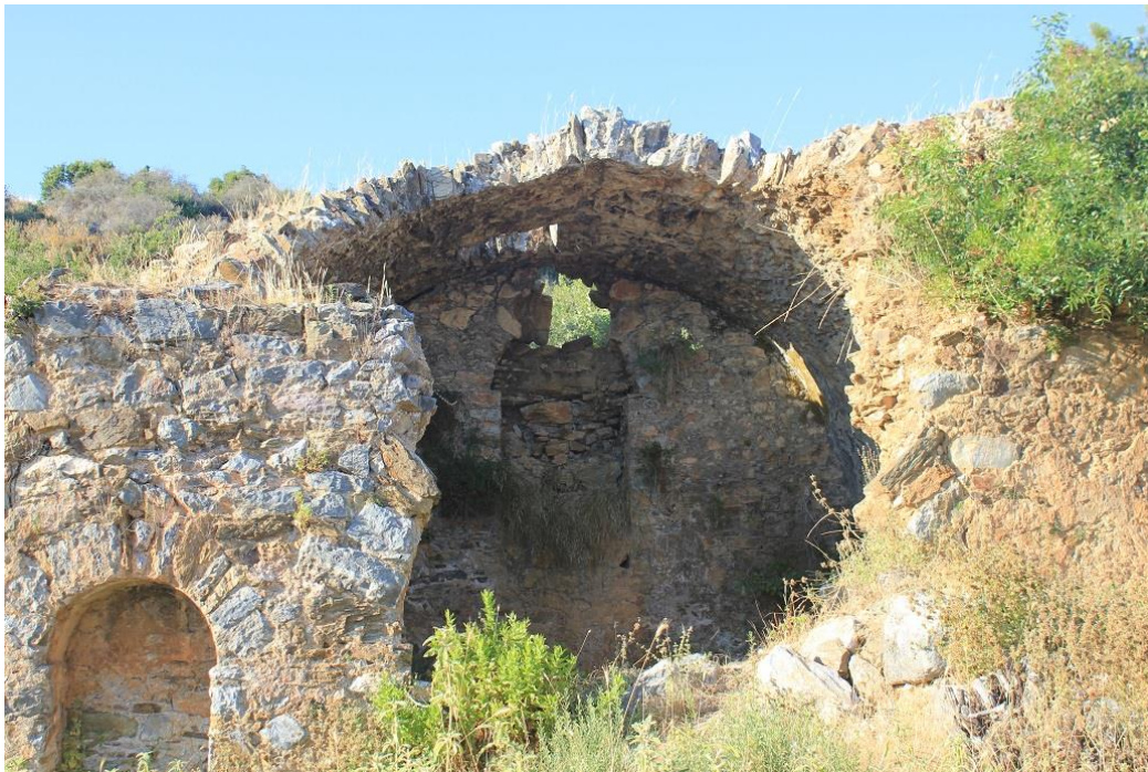
Figure 20: Partial view of Extramural Baths at Antiocheia ad Cragum, showing sub-ashlar masonry of the walls and partially preserved vault of radially laid uncut stone (photo by author).
