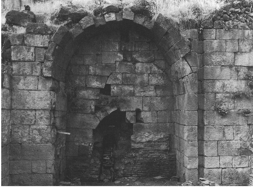
Figure 79: View of southern wall of the baths at Kanatha (modern Qanawat), showing basalt ashlar masonry (Peuser 2000, pl. 45c).
