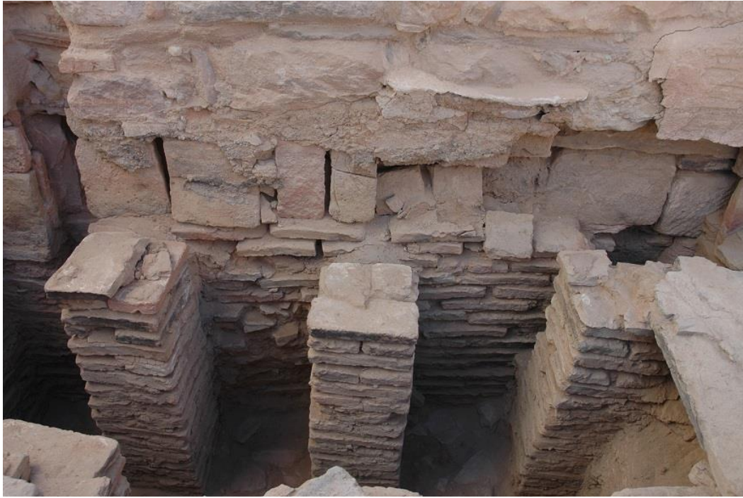
Figure 213: Close-up view of the hypocaust in Room D in the baths at Haurra (modern Humayma) (Reeves et al. 2017, fig. 17).
