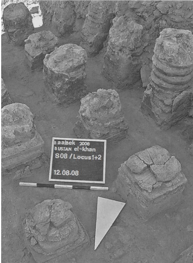
Figure 190: Close-up view of the hypocaust in the baths at Baalbek, showing use of square bricks in the pilae (Brünenberg 2009, Fig. 8).
