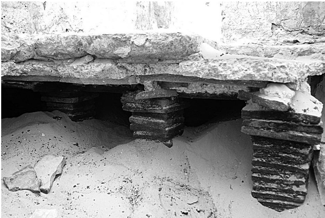
Figure 218: Close-up view of the hypocaust in the baths at Arieldela (modern 'Ayn Gharandal), showing use of square bricks in pilae and square capping bricks (Harvey 2019, fig. 10).
