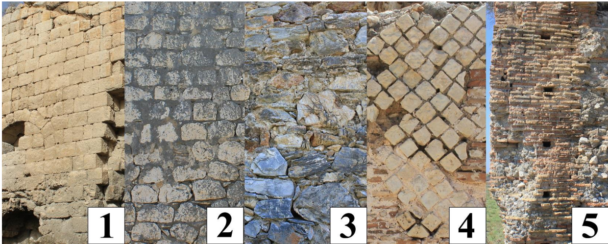
Figure 10: Examples of masonry techniques. 1 – ashlar; 2 – sub-ashlar; 3 – rubble; 4 – opus reticulatum ; 5 – brick (photos by author).
