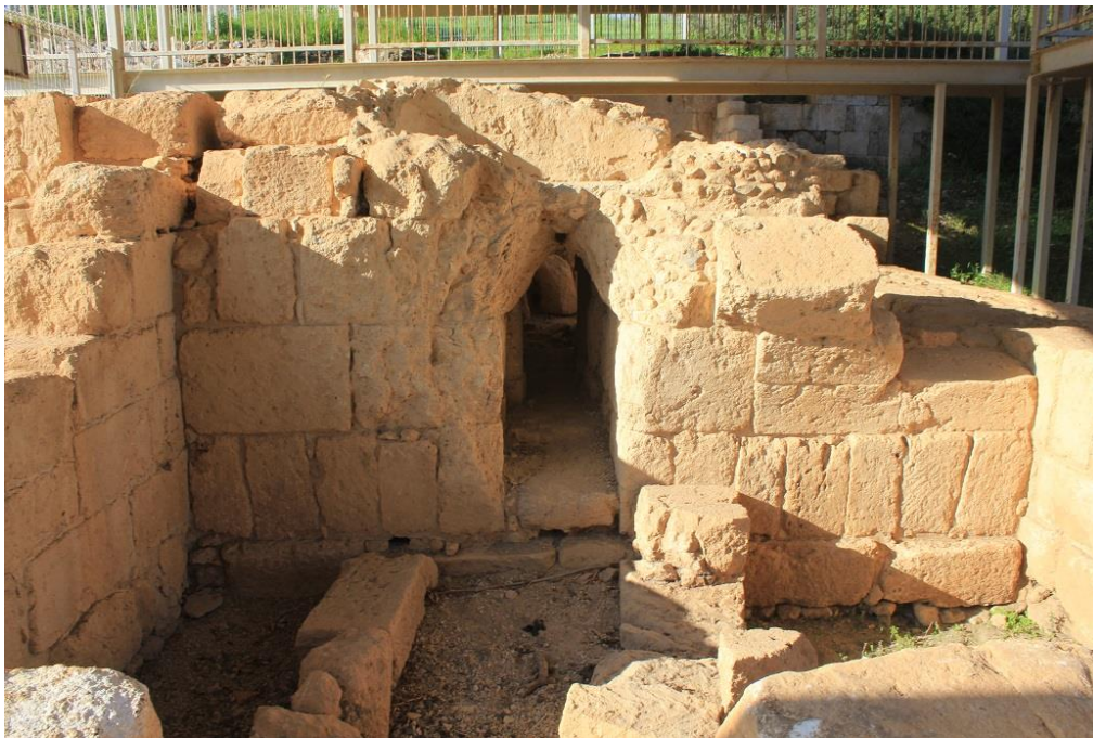
Figure 96: View of the praefurnium stoke hole in the baths at Ramat Hanadiv, showing limestone ashlar construction of the walls (photo by author).
