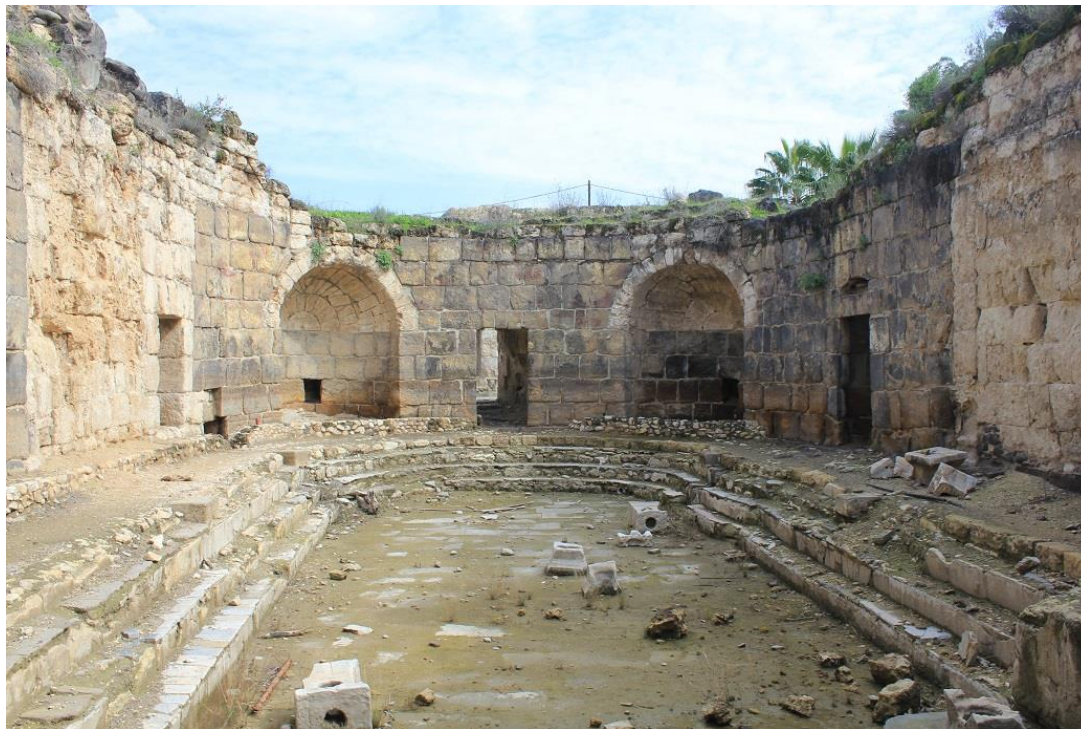
Figure 84: Interior view of the baths at Hammat Gader, showing use of both basalt and limestone ashlar construction (photo by author).
