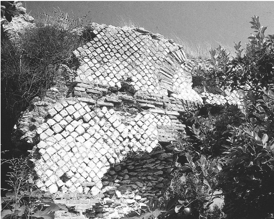
Figure 32: Detail of masonry of Reticulate Baths at Elaeussa Sebaste, showing use of opus reticulatum (Spanu 1999, fig. 54).
