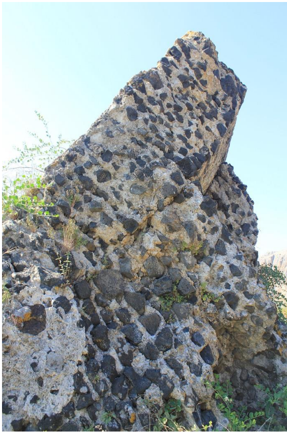
Figure 150: Large section of tumbled vaulting from the Southern Baths at Anazarbos, showing use of volcanic scoria as caementa in the mortared rubble (photo by author).
