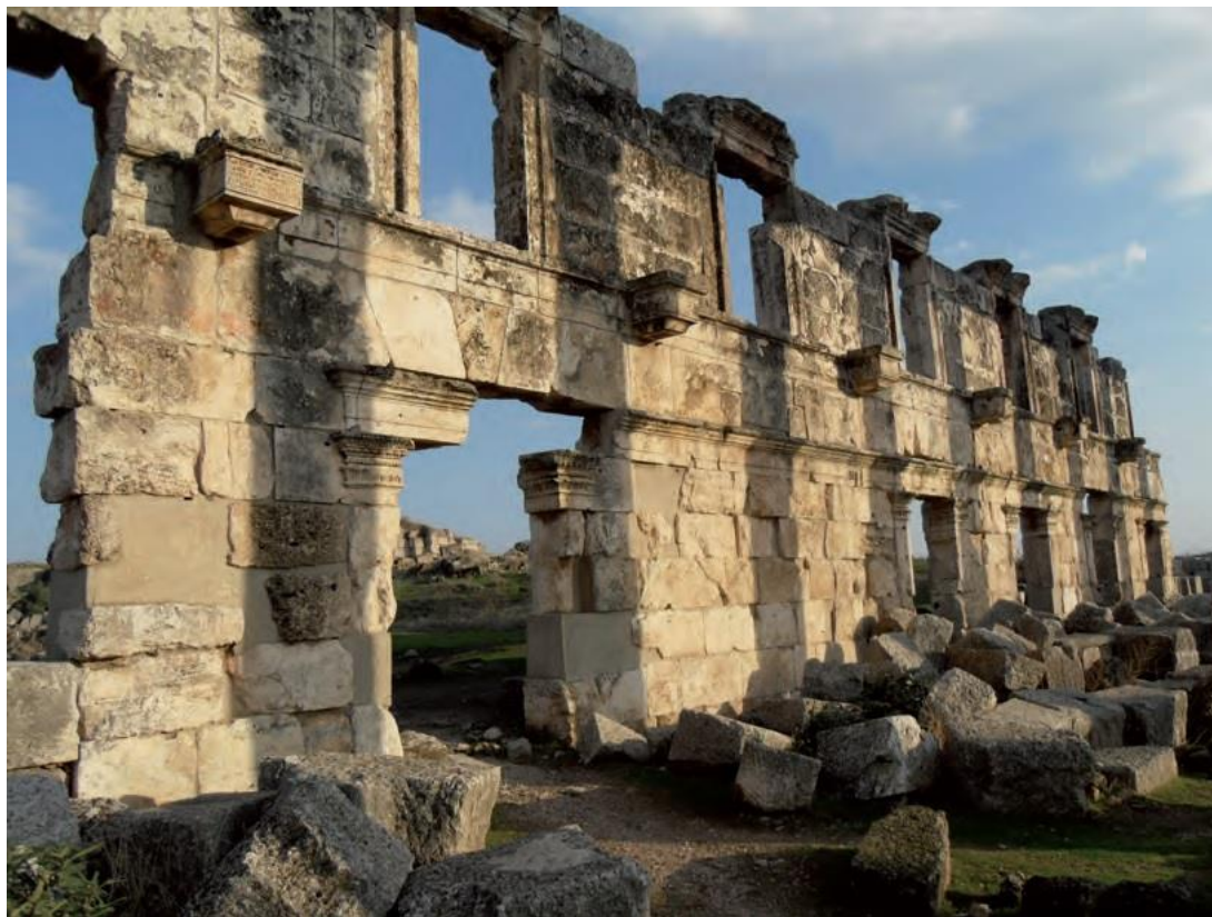
Figure 58: View of the Baths of L. Julius Agrippa at Apamea, showing limestone construction of back wall of eastern portico (Vannesse 2015, fig. 2).
