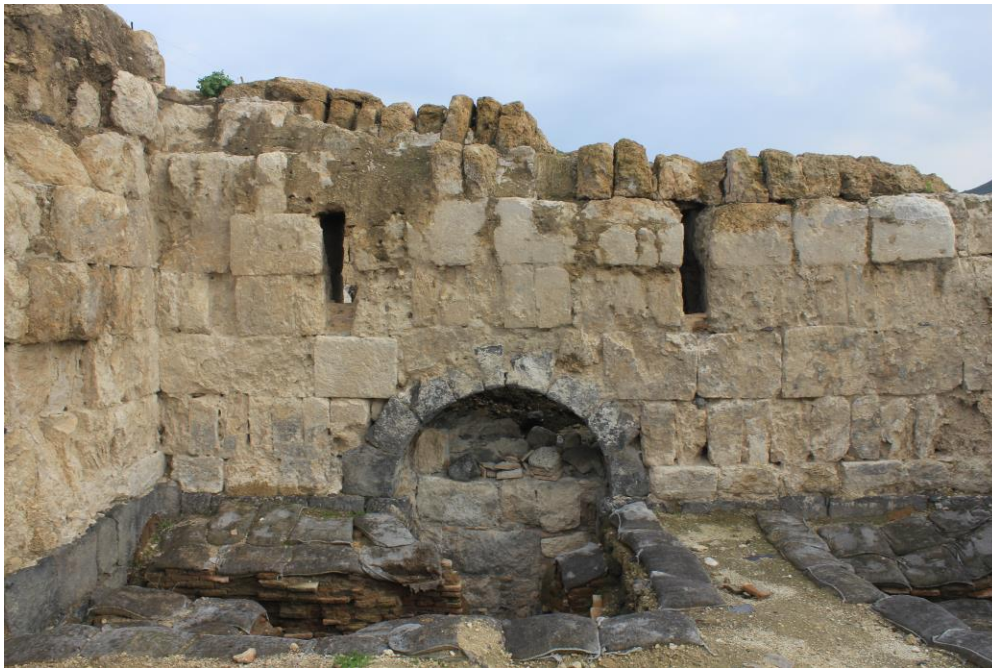
Figure 82: Interior view of heated room in the Southern Bathhouse at Hippos-Sussita, showing use of basalt ashlars in foundations (most visible in bottom left of image) and limestone ashlars set in isodomic courses alternating between headers and stretchers (photo by author).
