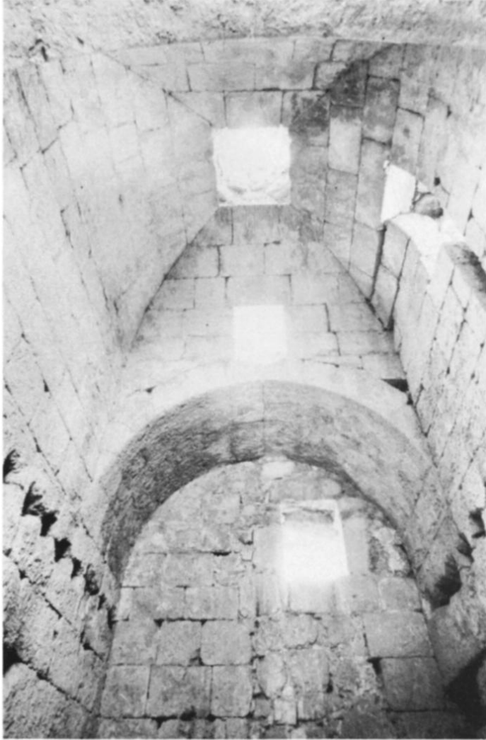
Figure 105: Interior view of Room 4 in the baths at Emmaus, showing ashlar masonry and ashlar vaulting (Gichon 1979, pl. 12a).
