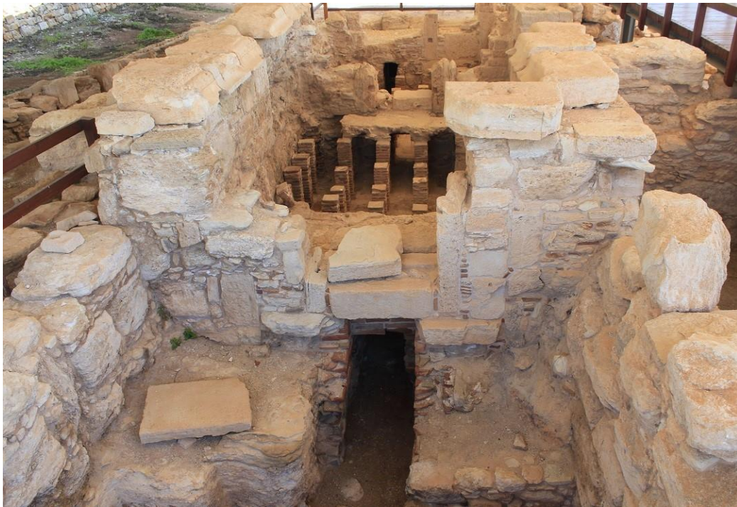
Figure 48: View of baths at the Sanctuary of Apollo Hylates, with prae-furnium in foreground, showing masonry of unfinished blocks of ashlar mixed with rubble (photo by author).
