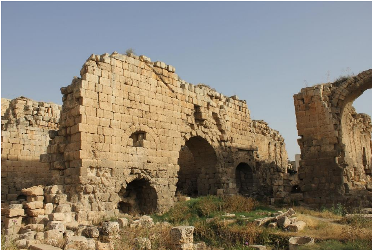
Figure 115: View of the East Baths at Gerasa (modern Jerash), from northwest, showing ashlar masonry (photo by author).
