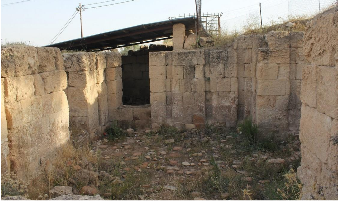
Figure 122: Interior of Room 6 in the baths at Birketein, showing ashlar masonry. In the far wall it is possible to see the vertical grooves for flue vents and vertically placed square bricks at base of wall for lining the hypocaust (photo by author).
