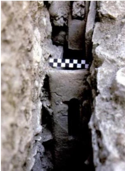
Figure 181: Close-up view of slab-made tubulus in the Harbor Baths at Elaeussa Sebaste (Borgia and Spanu 2003, fig. 246).
