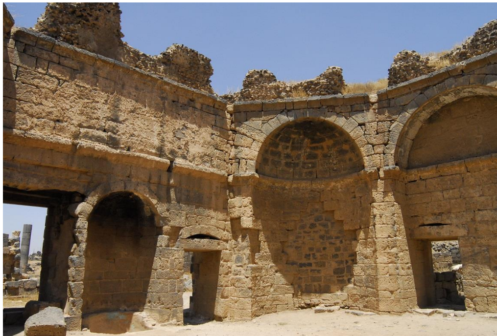
Figure 109: Interior view of the frigidarium of the South Baths at Bosra, showing basalt ashlar masonry and mortared rubble vaulting using scoria for caementa (photo by author).
