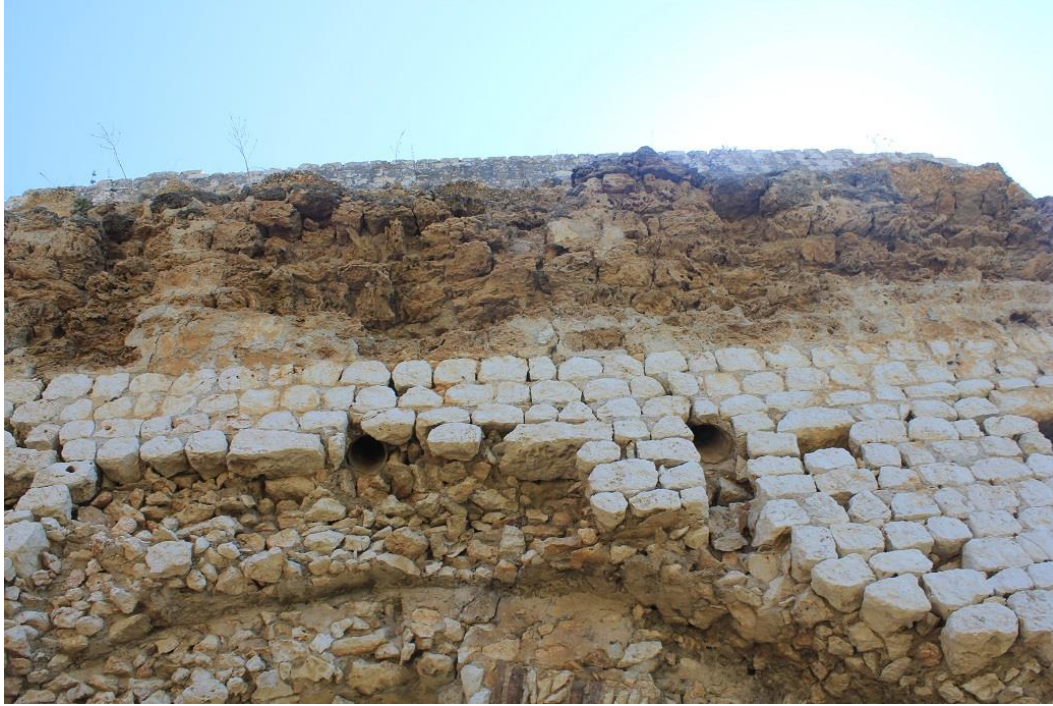
Figure 29: Detailed view of the Large Baths at Elaeussa Sebaste, showing sub-ashlar masonry, mortared rubble core, and tufa blocks in remains of vault (photo by author).
