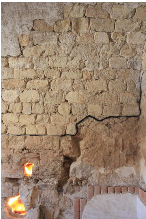
Figure 166: Interior view of the caldarium in the Large Baths at Masada, showing reconstructed vault of stone blocks (masonry below black line is original) (photo by author).
