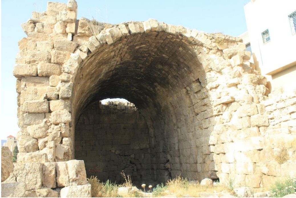
Figure 168: View of the East Baths at Gerasa (modern Jerash), showing the intact ashlar vaulting (photo by author).
