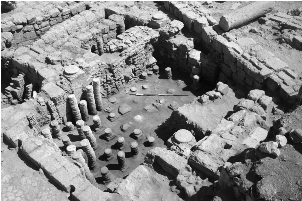
Figure 208: View of the hypocaust in Room C1 in the Central Baths at Gerasa (modern Jerash) (Blanke 2015, fig. 3).
