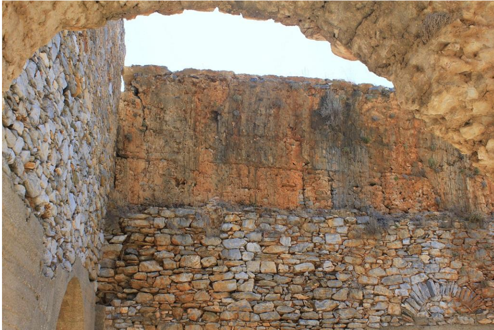
Figure 24: View of interior of Bath III 2 B at Anemurium, showing the use of roughly dressed quarried limestone in walls and mortared rubble packing above brick intrados that still preserves impressions of the vertically placed bricks, now fallen away (photo by author).
