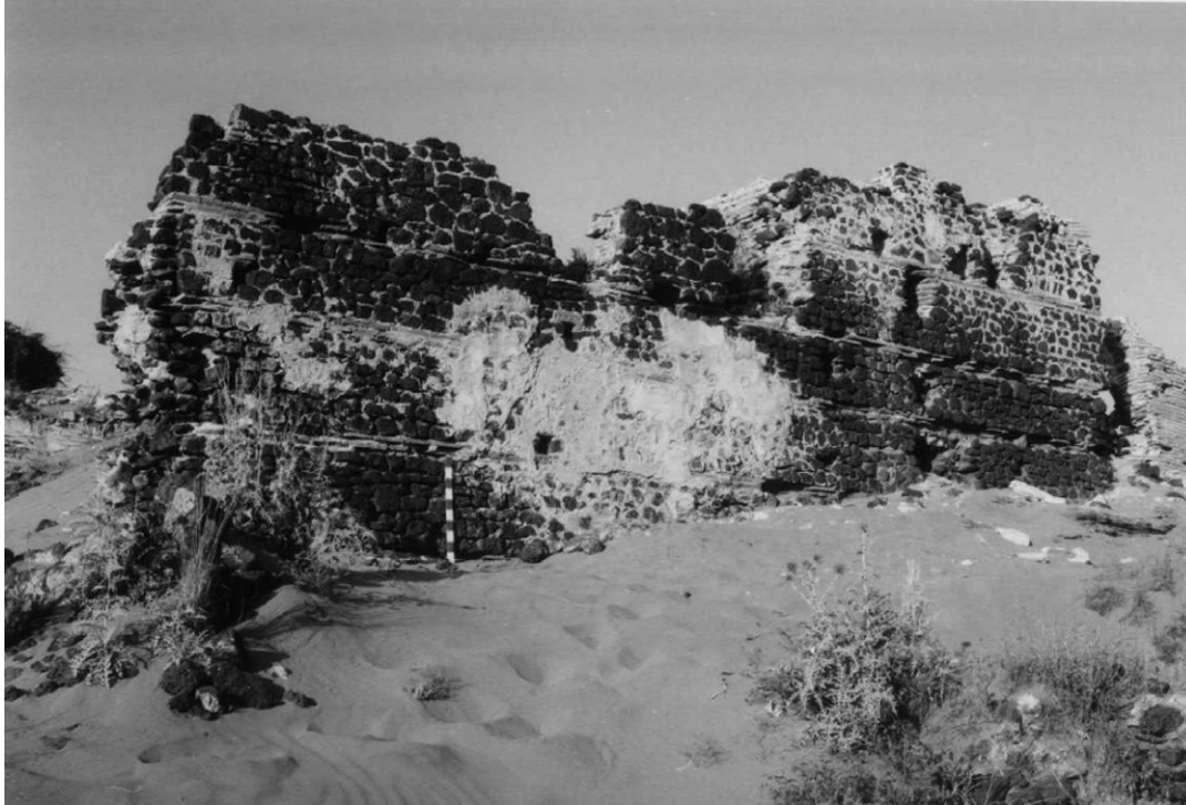
Figure 40: View of north wall of the Larger Baths at Küçük Bernaz, showing use of carefully shaped polygonal basalt stones (Tobin 2004, fig. 56).
