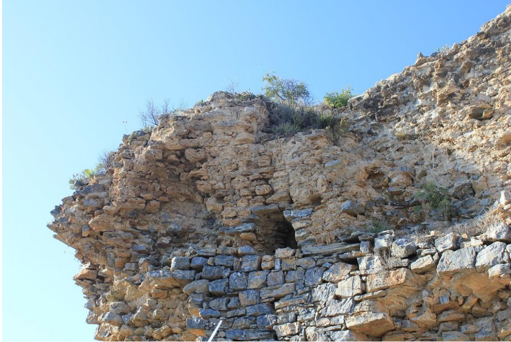
Figure 17: View of vaulting in Room 8 of Great Baths at Antiocheia ad Cragum, showing sub-ashlar masonry of wall and lime-tufa blocks of vaulting (photo by author).
