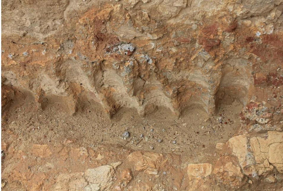
Figure 217: Close-up view of mortar impressions of cylindrical heating pipes against wall of heated room in baths at Tamara (modern En Hazeva) (photo by author).
