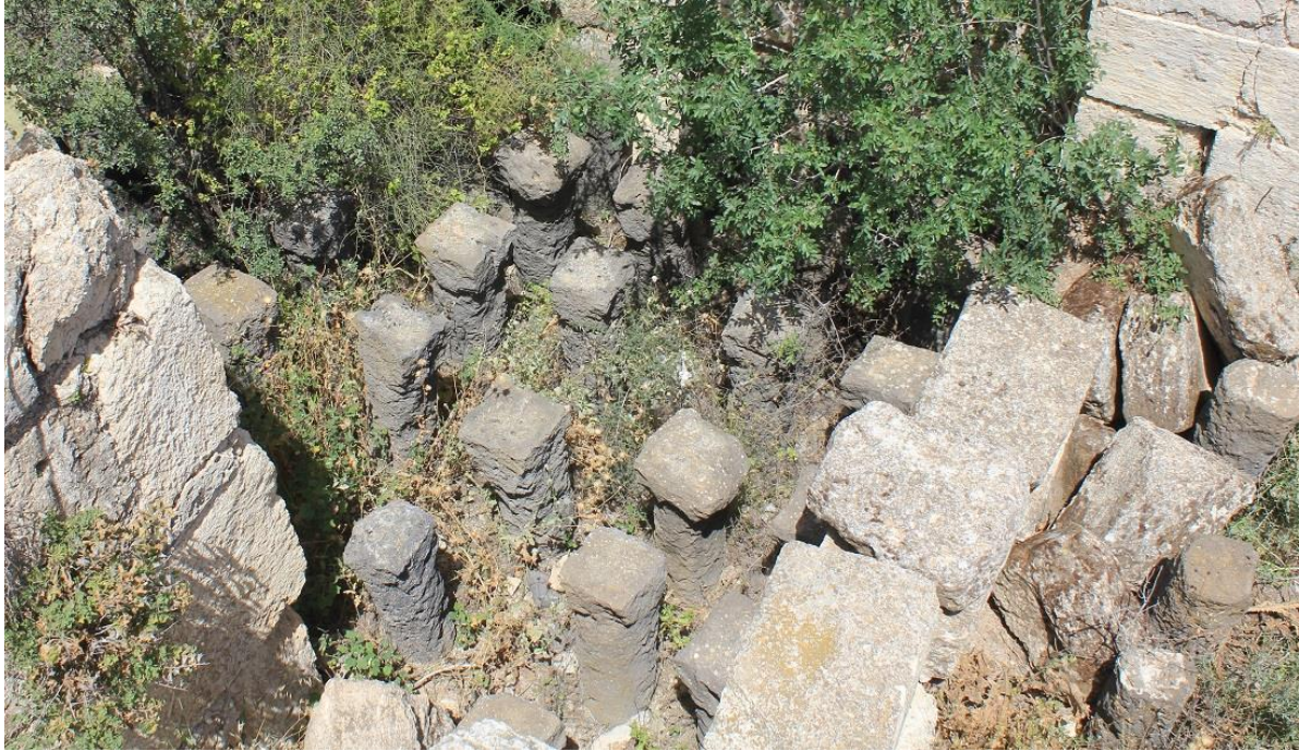
Figure 194: View of basalt pilae in the hypocaust of the Byzantine Baths at Gadara (modern Umm Qais) (photo by author).
