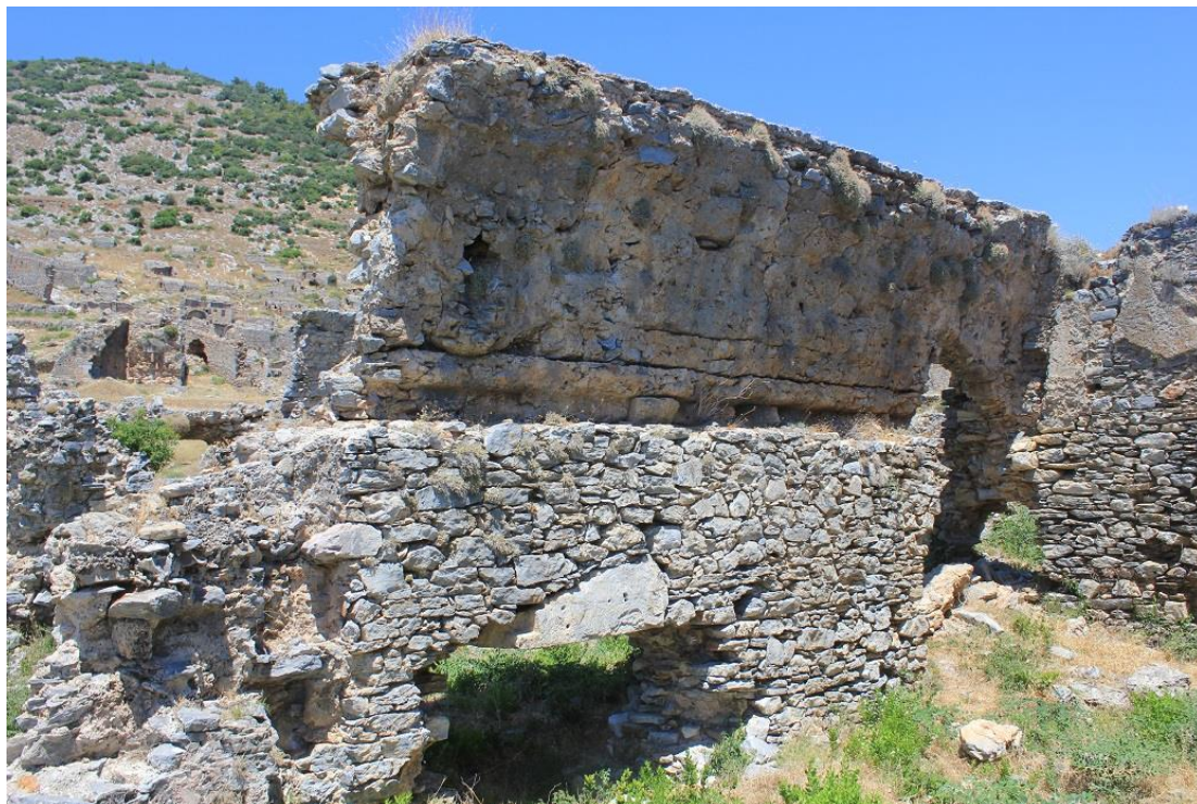
Figure 26: View of Bath II 11 B at Anemurium, from southeast, showing use of irregular limestone in the masonry of the walls (photo by author).
