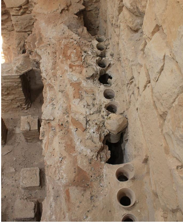
Figure 223: Close-up view of cylindrical heating pipes in situ in the baths at Oboda (modern Avdat) (photo by author).
