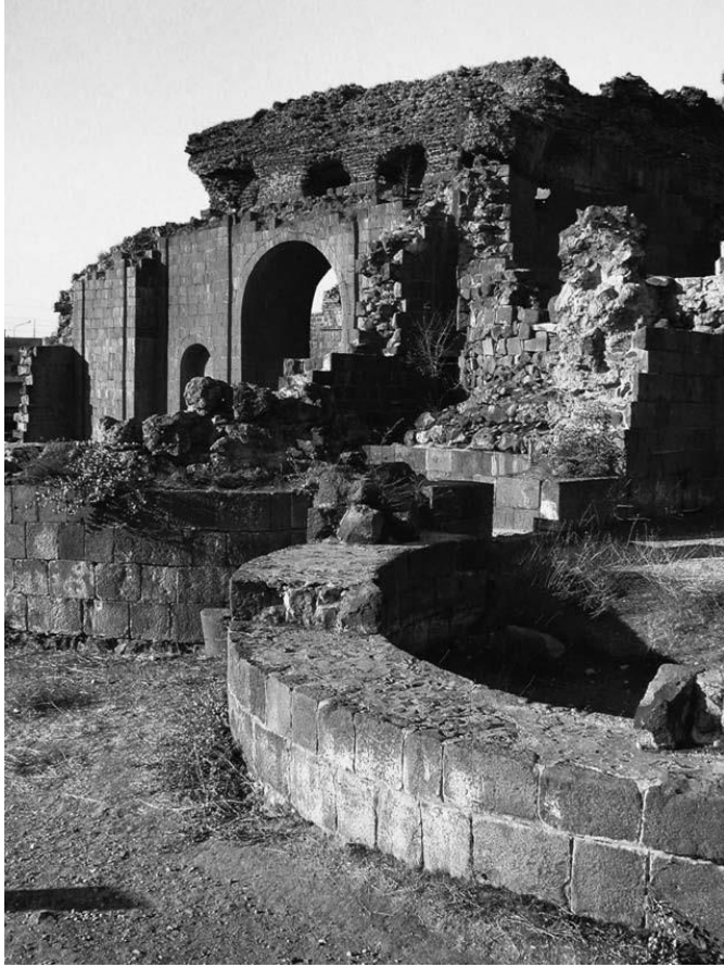
Figure 75: View of the baths at Philippopolis (modern Shahba), from west, showing basalt ashlar masonry and remains of scoria vaulting above (after Fournet 2012b, fig. 12).
