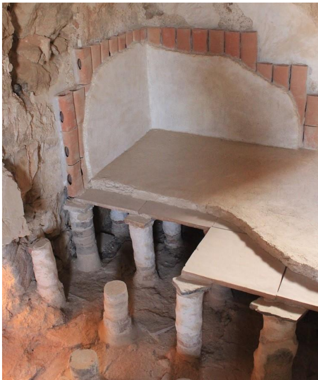
Figure 8: Reconstruction of hypocaust and wall-heating system in Large Baths at Masada, showing raised floor supported by pilae and tubuli against walls (photo by author).
