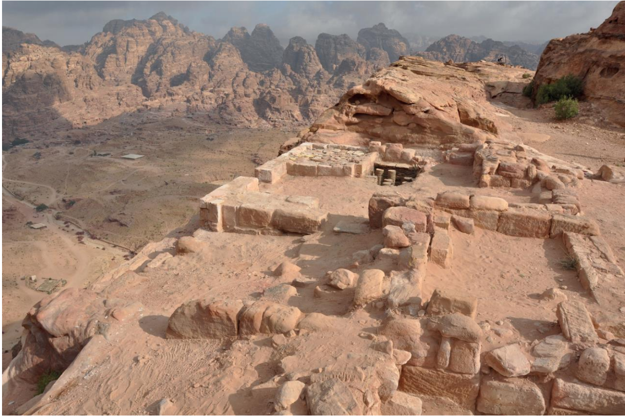
Figure 128: View of baths on Jebal Khubthah, overlooking Petra, showing use of sandstone ashlar masonry (Fournet and Paridaens 2016, fig. 11).
