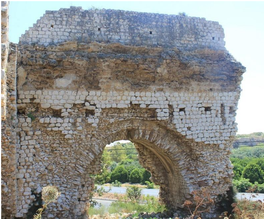
Figure 28: View of the Large Baths at Elaeussa Sebaste, showing sub-ashlar masonry, mortared rubble core, and tufa blocks in remains of vault (photo by author).
