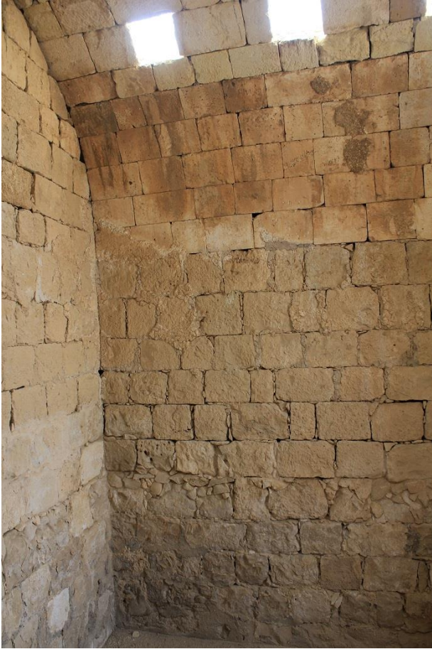
Figure 136: Interior of the baths at Oboda (modern Avdat), showing ashlar masonry of the walls and vault (photo by author).
