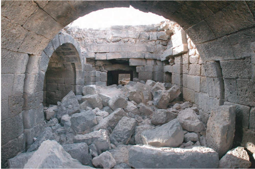
Figure 73: Interior of caldarium in the baths at Sha'arah before excavation, showing basalt ashlar construction (Fournet 2008a, fig. 9).
