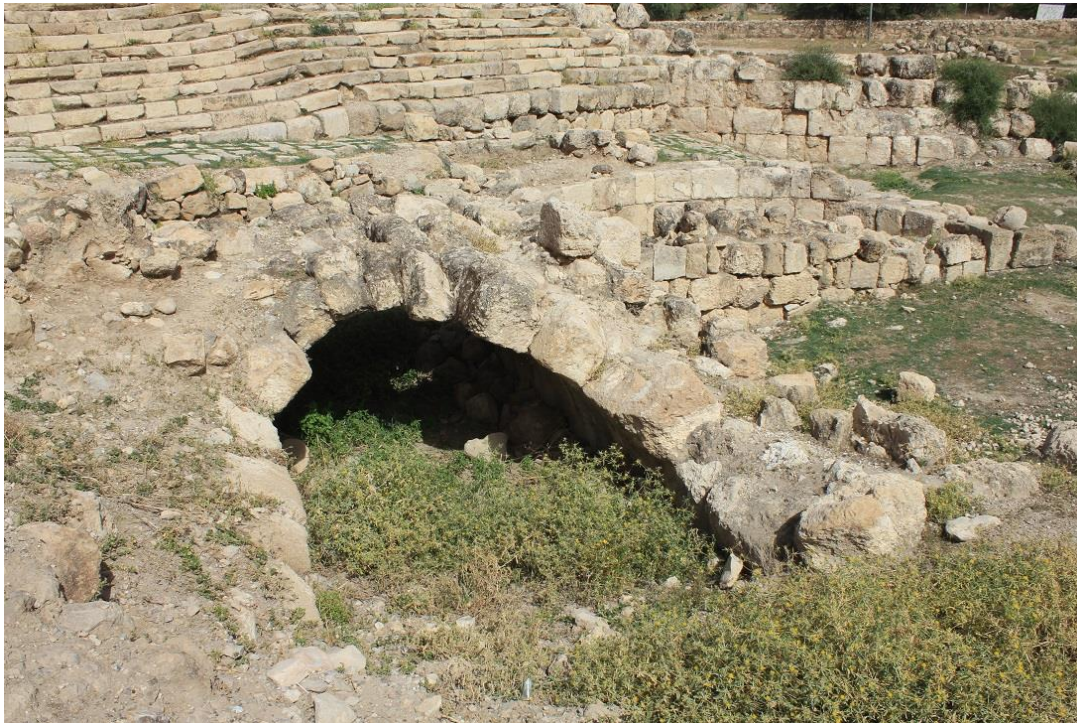
Figure 162: View of the baths at Pella, showing ashlar vaulting (photo by author).
