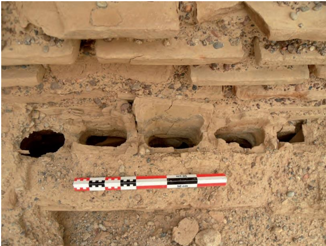
Figure 189: Close-up view of in situ tubuli in Bath E3 at Dura Europos (Vannesse 2015, fig. 12).
