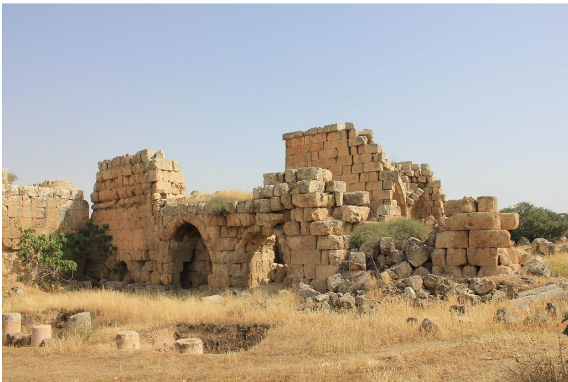
Figure 117: View of the West Baths at Gerasa (modern Jerash), from north, showing ashlar masonry (photo by author).
