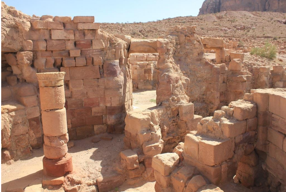
Figure 126: Interior view of baths next to the Petra Great Temple at Petra, showing sandstone ashlar masonry (photo by author).
