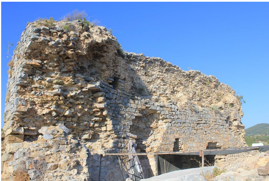
Figure 16: View of Room 8 of Great Baths at Antiocheia ad Cragum, from west, showing sub-ashlar masonry (photo by author).
