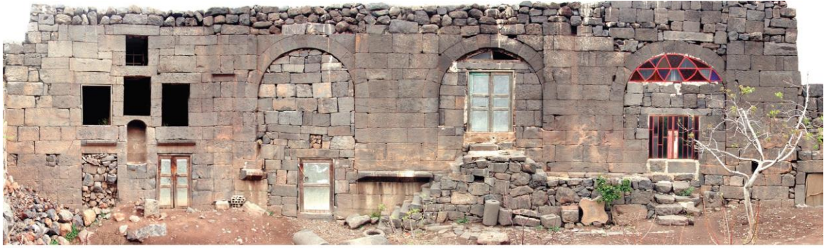
Figure 77: Southern façade of the baths at Selaema (modern Salim), showing basalt ashlar masonry (after Fournet 2010, fig 2).
