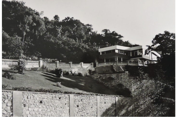
Figure 1-12 Residence, R. Malbranche, Port-au-Prince, c. 1970 (personal papers)
