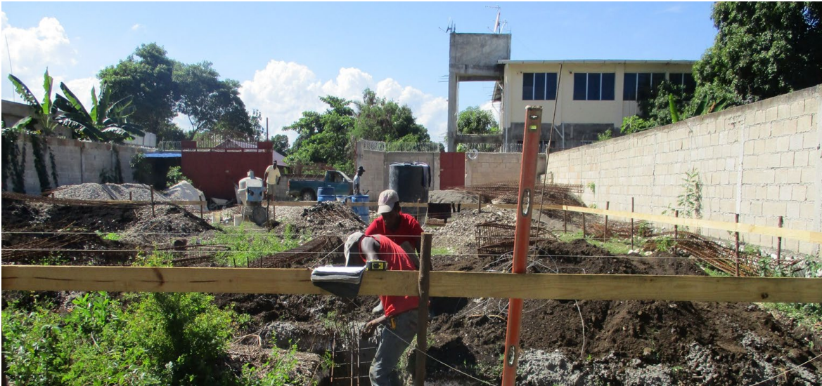
Figure 4-1 Workers excavating foundation trenches at Chantye Divisyon, Leyogann, Haiti 2018
