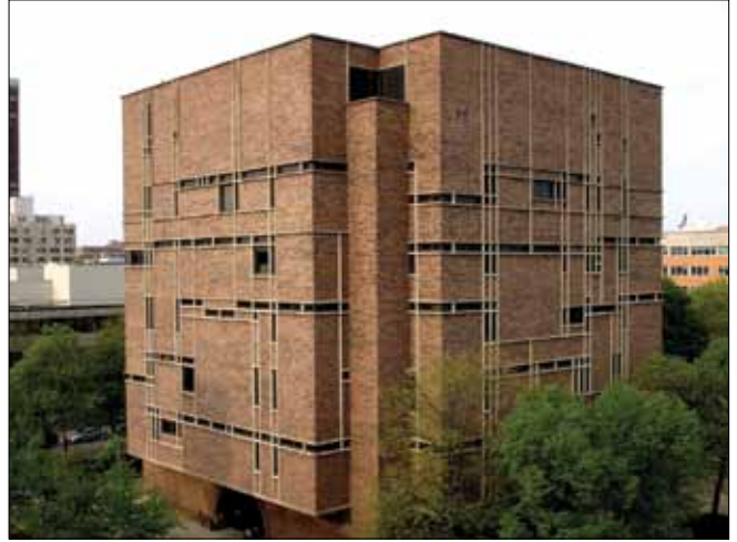
Fleming Administration Building
