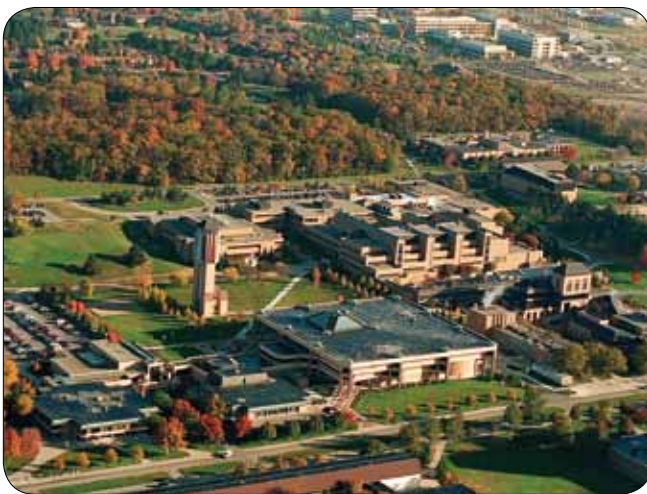
2000s The Engineering Campus is complete.
