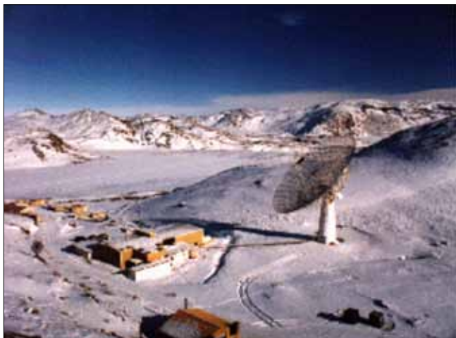
Radar Installations for UARC Collaboratory
