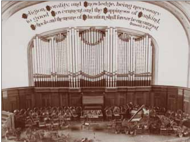
The words of the Northwest Ordinance in the auditorium of old University Hall
