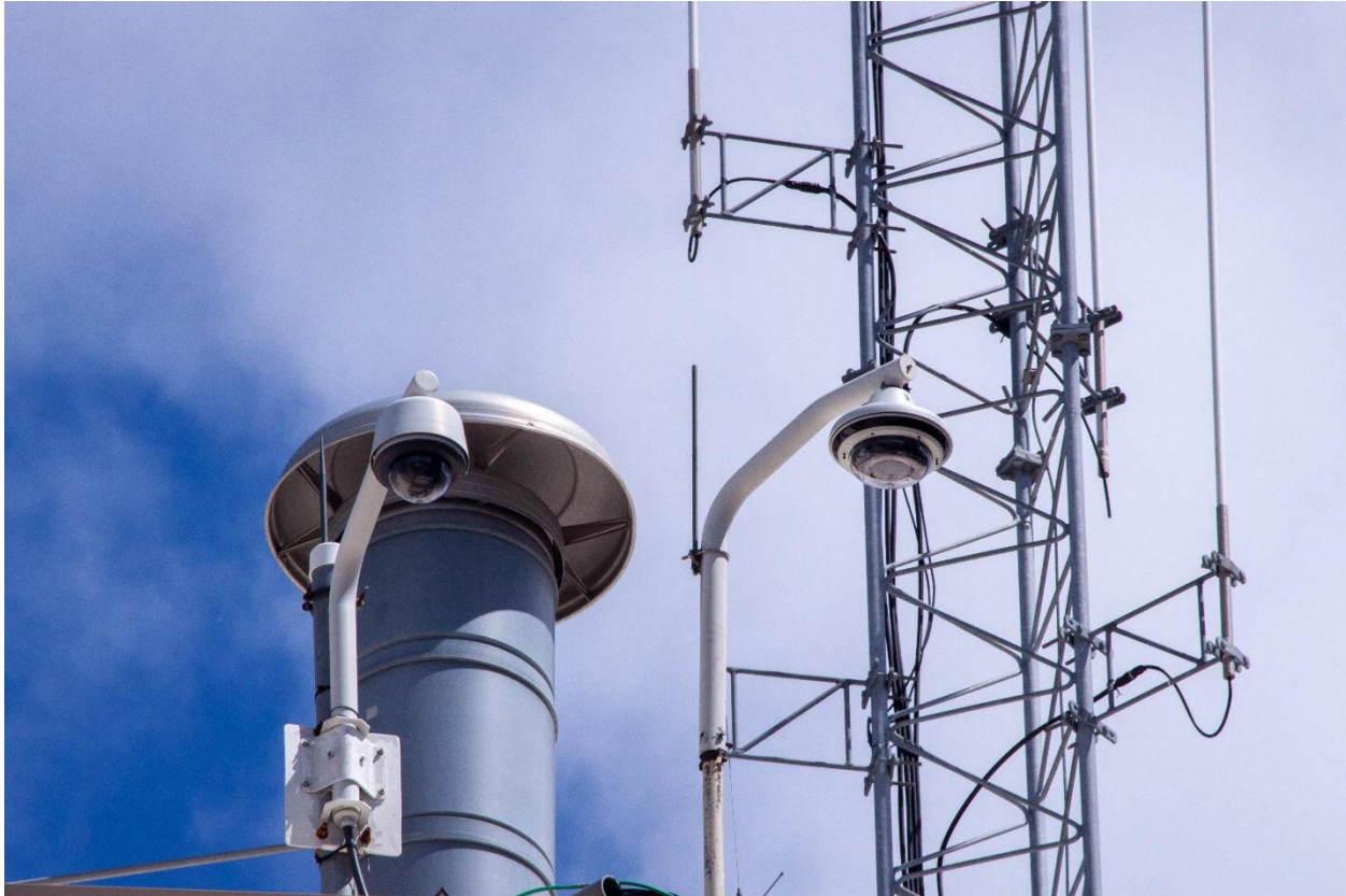
Figure 5. A photograph of two cameras placed on the roof of the station: Hudson, Craig. 15 April 2021.
