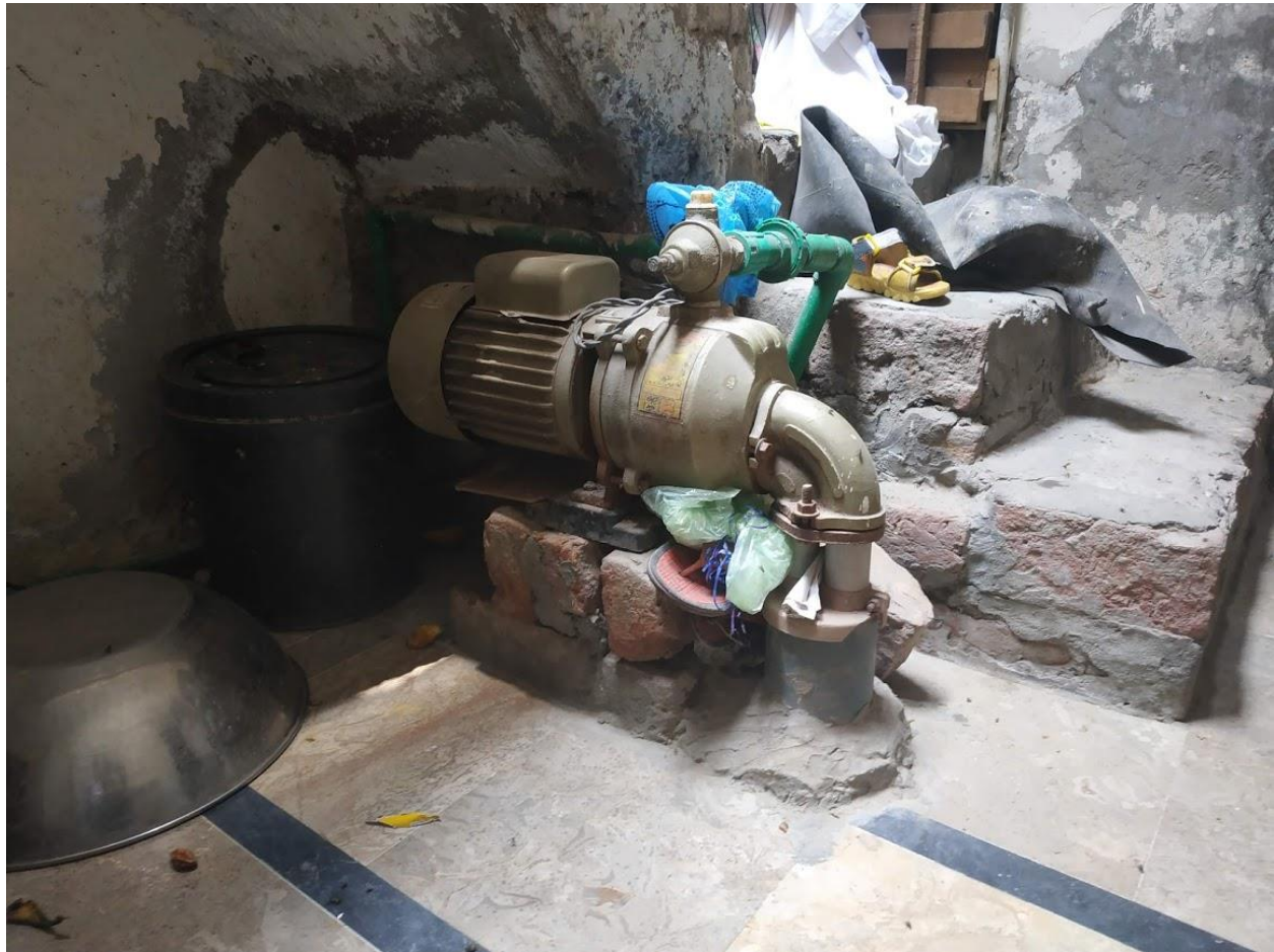
Fig 1: Electric water pump connected to a borewell installed inside an interviewee's home. Pumps were generally run once a day, often in the mornings siphoning water into large storage tanks on the roofs of families' homes.
