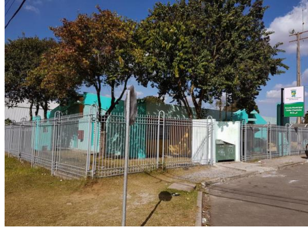
Figure 1.10: School Built Adjacent to Vila Governador 40
