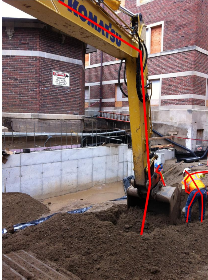
Figure 2.1 Illustration of the 2D Pose Estimation System on a Video Frame for Both Articulated Construction Robot and Human Workers.
