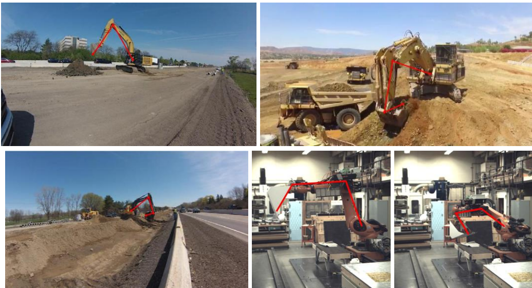
Figure 2.17 Results of the Excavator 2D Pose Estimation.
