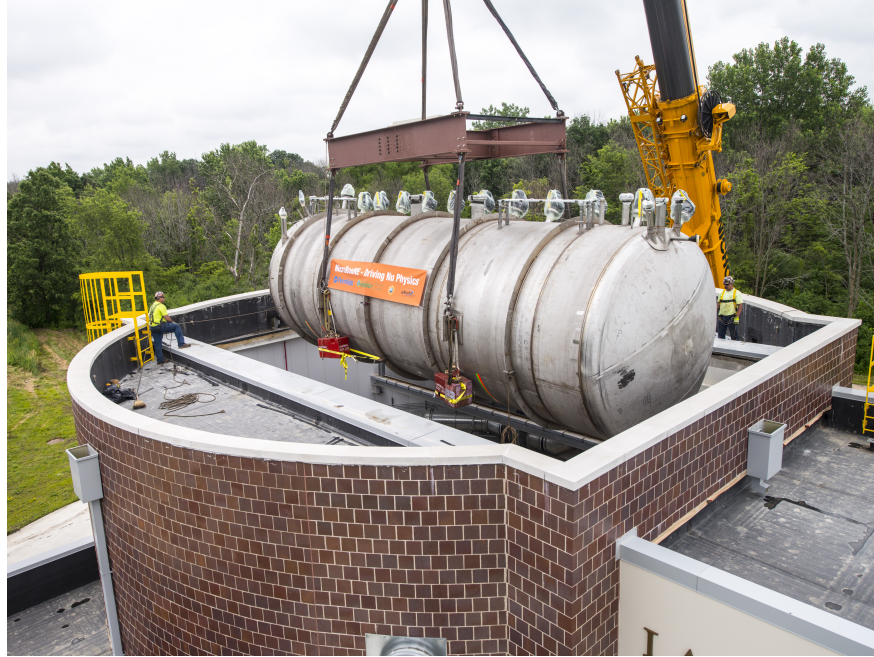
Figure 5.1: The MicroBooNE detector being lowered into the detector hall at Fermilab. Courtesy of Fermilab.
