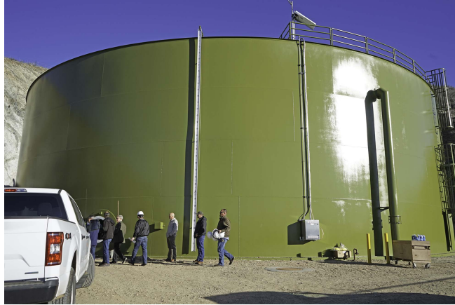
Figure 11. Prescott Valley water tank that can hold 2 million gallons of water [22]
