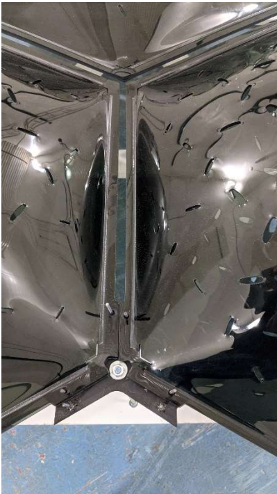
Figure 6 – Detail of air gaps between adjacent pairs of glass plates
