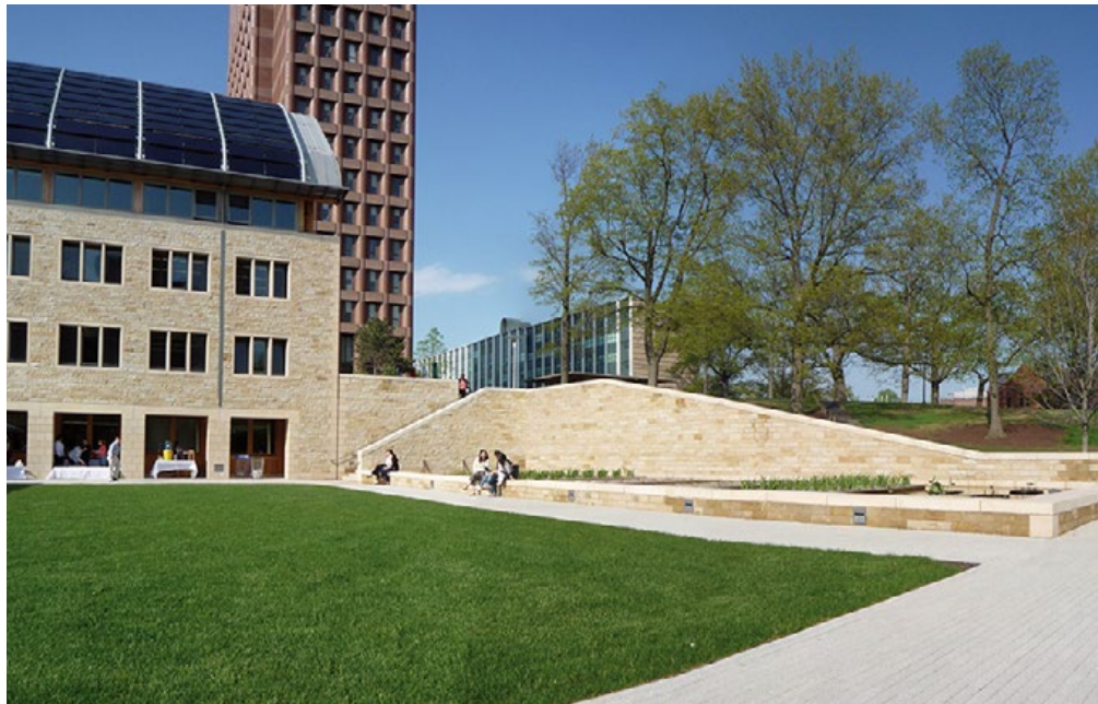
Completed design at Kroon Hall, Yale University 19
