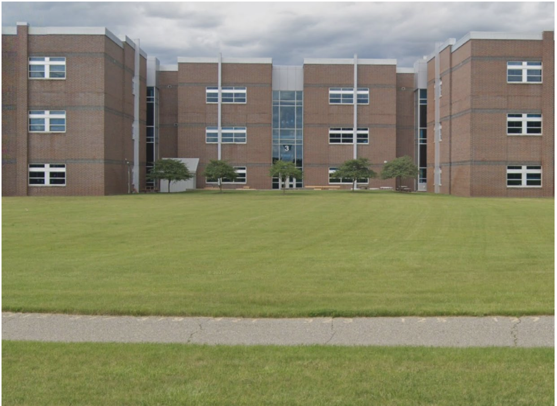
▲ Existing condition; Photo: Google
