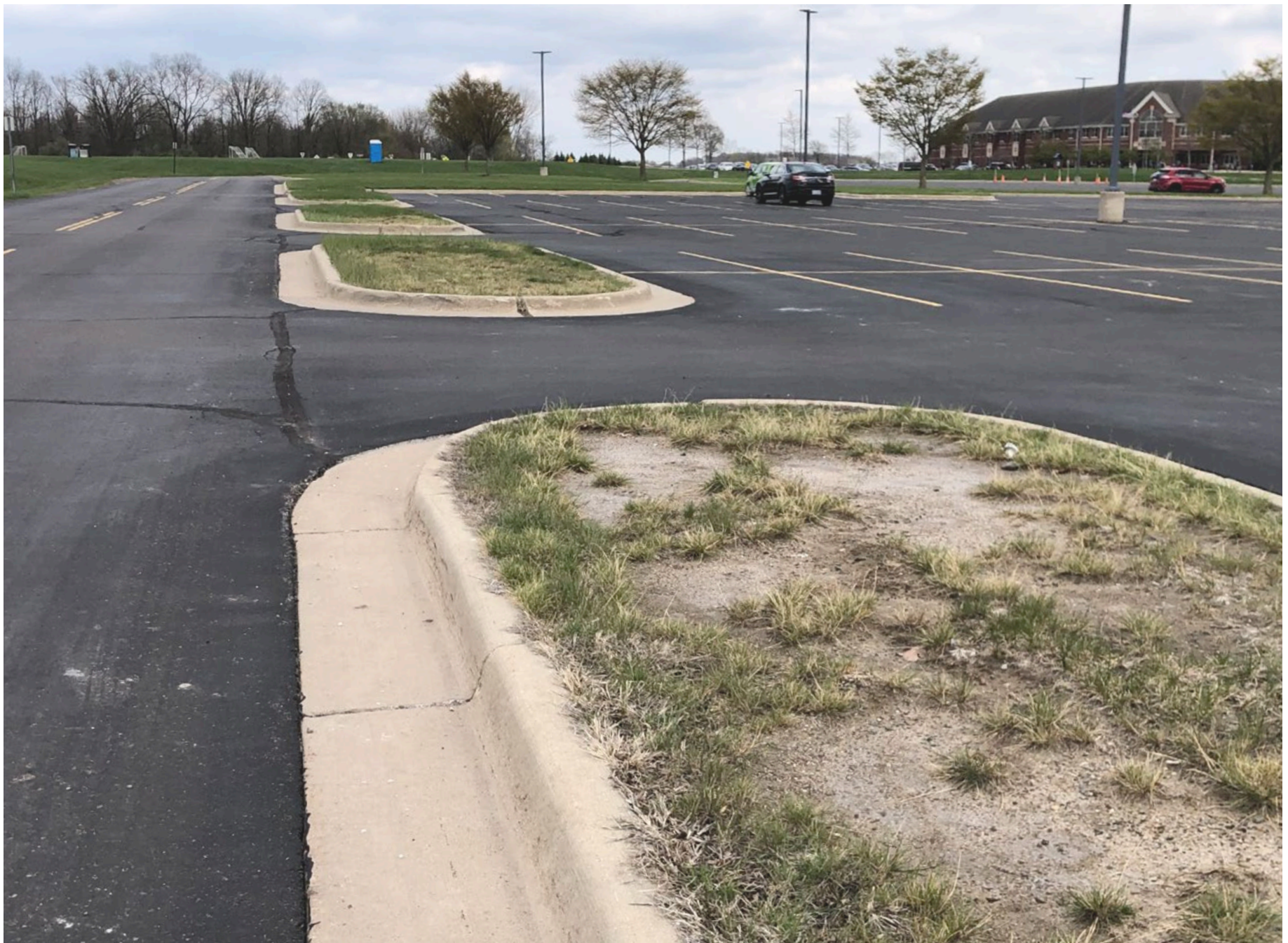
▲ Existing condition; Photo: Emily Hernandez
