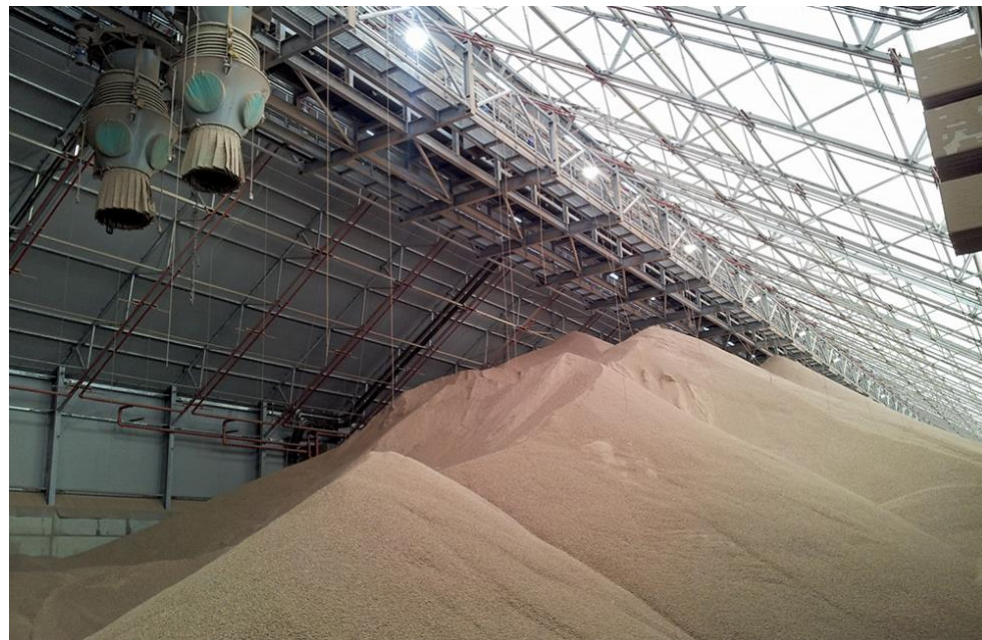
Biomass Facilities Buildings
