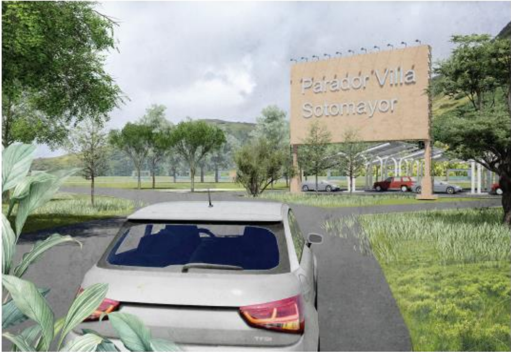
Main Entrance. Solar Carport
