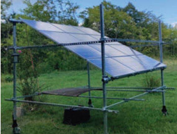
Large Stilt Structure (Steel or Wood)
