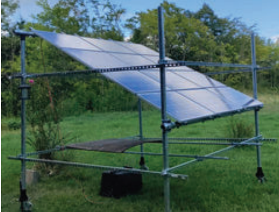
Large Stilt Structure (Steel or Wood)
