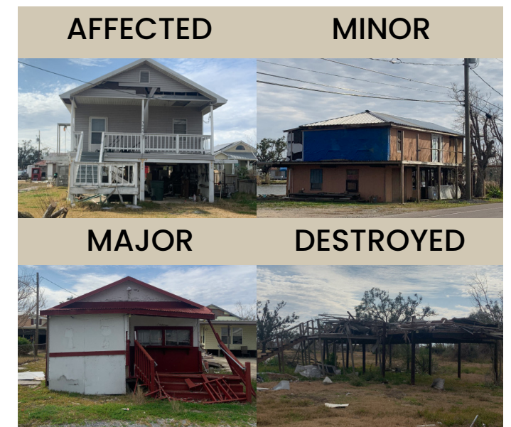
Image 2.4: FEMA PDA Categories:: There are four categories that classify severity of damage. Credit to Federal Emergency Management Agency.
