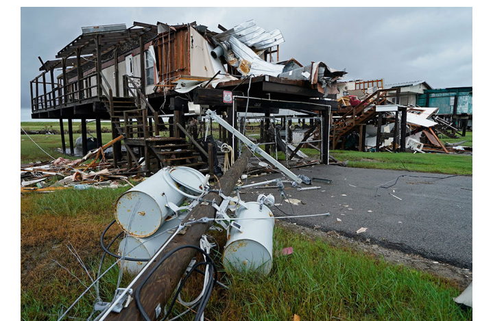
Image 1.2: Street-level imagery of disaster damaged stilted homes
