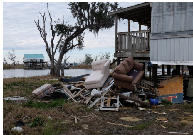
Image 2a.1: Debris Clearance in Southeastern Louisiana. This image demonstrates how perishable data is ripe only in short periods of time. In a few weeks, these debris piles that demonstrate community damage may be cleared, and destruction data eliminated. Machine learning can assist with the capture of data, but researchers should remember the evolution of data prevalence.
