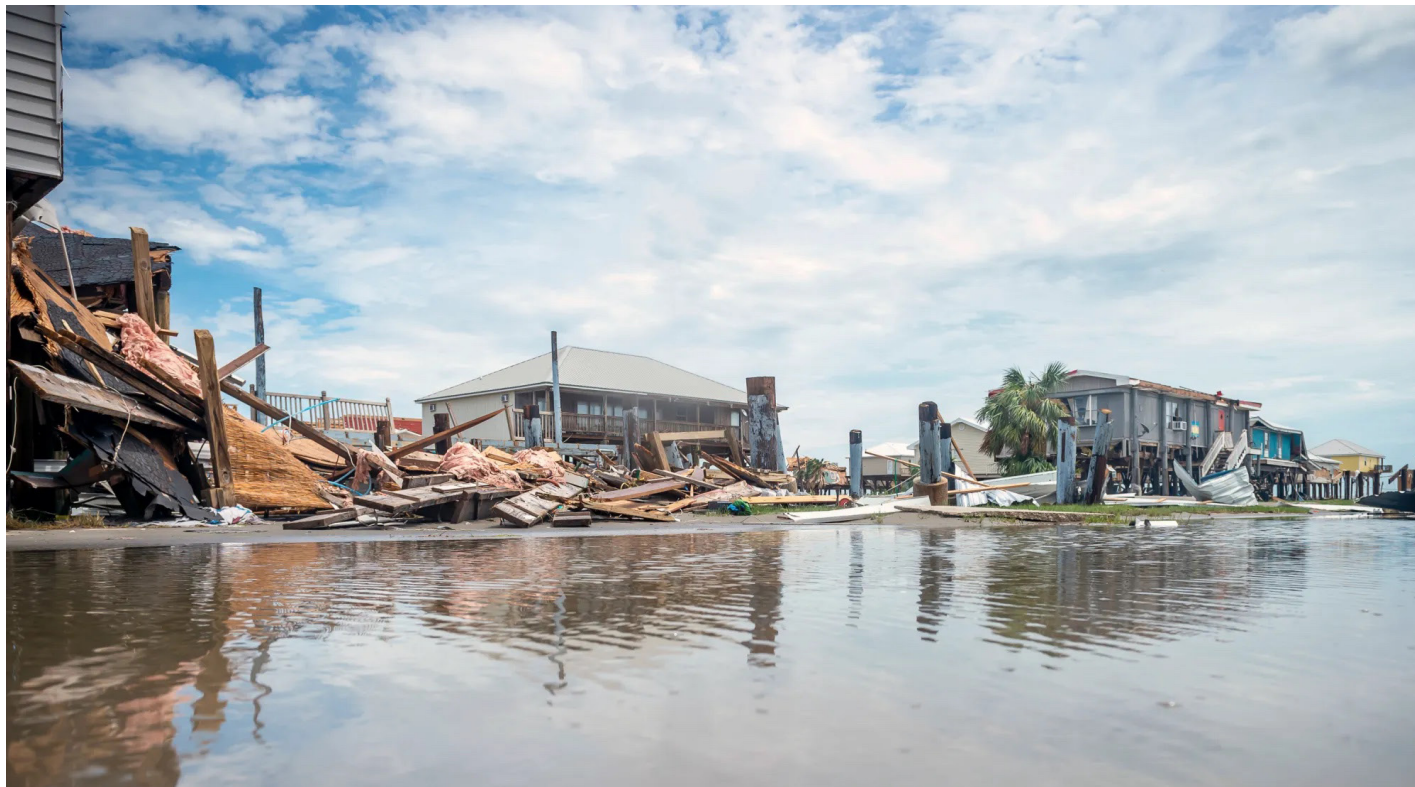
Image 1.4: Street-level imagery of disaster damaged homes
