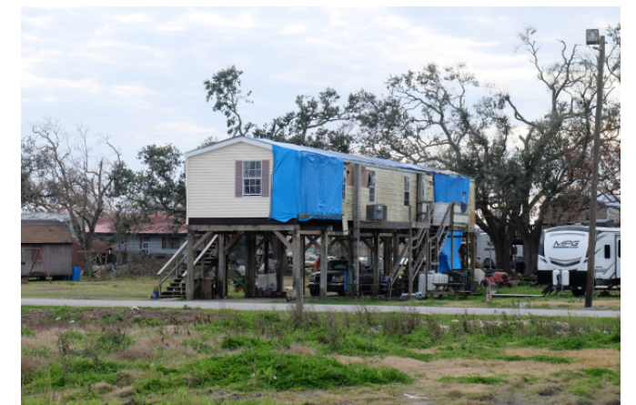
Image 2.1: A manufactured home in Dulac, Louisiana damaged from Hurricane Ida
