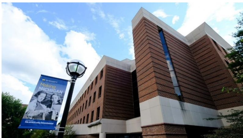
Figure 5.1. Chemistry building at the University of Michigan
