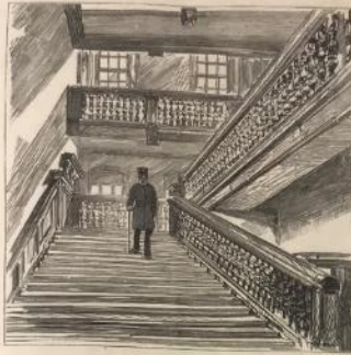
STAIRCASE TO WARDS
