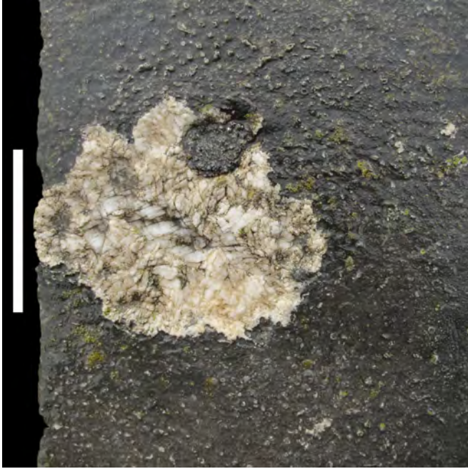
FIGURE 2 — Detail of the coping stone, a highly fossiliferous Mississippian limestone. The lobate mass of white calcite crystals, left of center, was presumably organic in origin, but is now unidentifiable. After slabbing, it was bored, but this hole is now infilled with cement. Syringopora sp. is prominent towards the top. Scale bar represents 50 mm.
