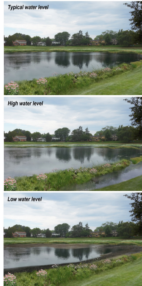
Figure 2.1 An example of sNBS: a retention pond in a residential area that is managed by a smart stormwater system. The pond was depicted with different water levels: 1) typical, 2) low, as if the pond were drained 24 hours before a storm to free up storage capacity, and 3) high, as if water were retained at a higher than the typical level for as long as 48 hours after a storm (visualizations by Yiiran Shen and Yuanqiu Feng).
