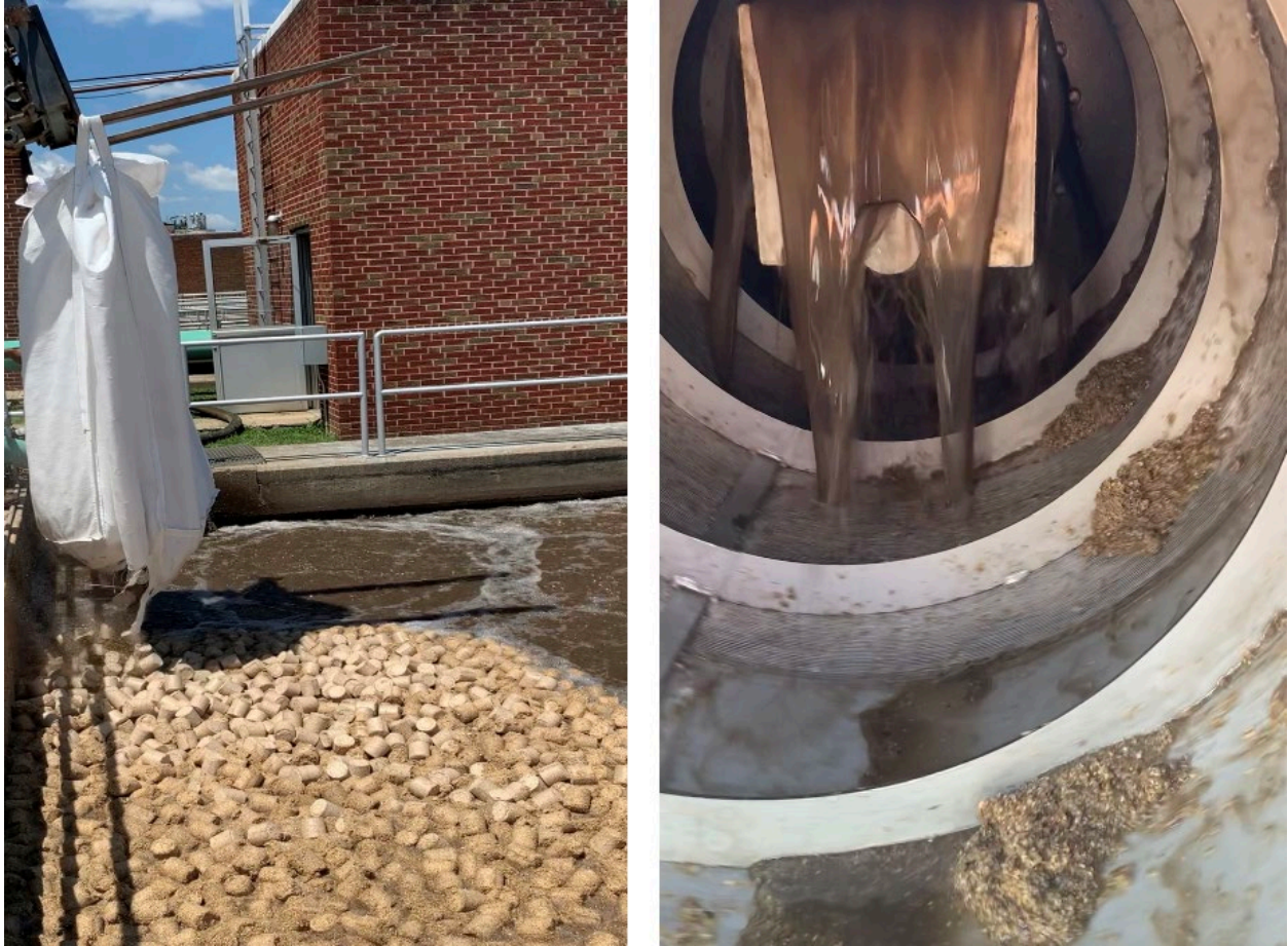
Figure 1. (left) Mobile-biofilm carriers (i.e., kenaf) are compressed and packed in sacks and are easily integrated with an existing WWT process. (right) Mobile-biofilm carriers are retained by screens, discharged into a sump, and flow with screen wash water into a location selected for their re-introduction to a WWT process.
