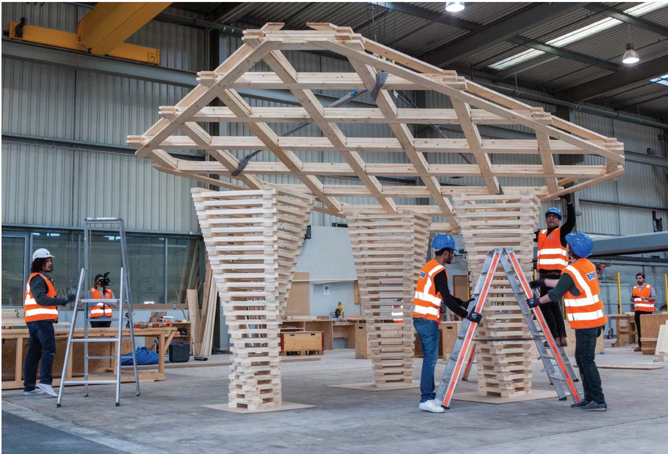
6 Connecting the pre-assembled roof and vertical supports
